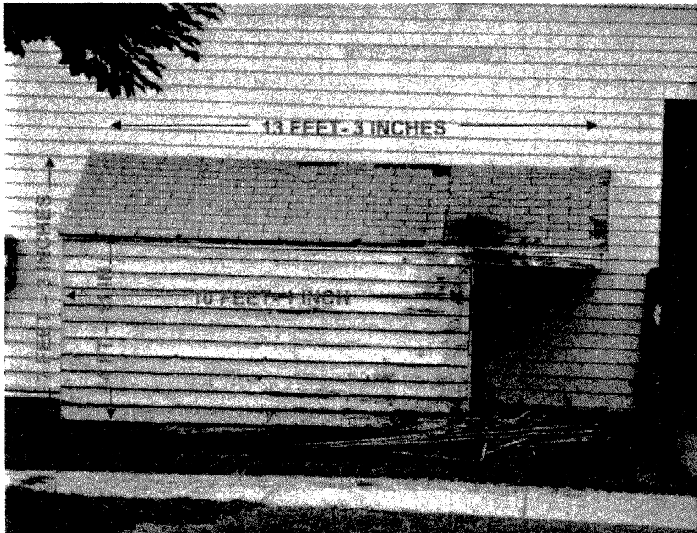
Close Up Picture Of Attached Shed
