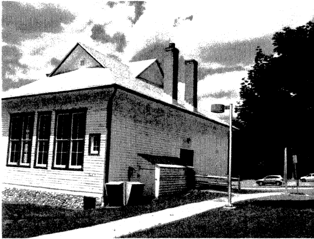
Rear of Historic Clarksburg School Showing Attached Shed
