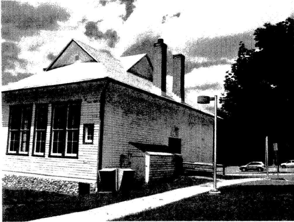
Rear of Historic Clarksburg School Showing Attached Shed
