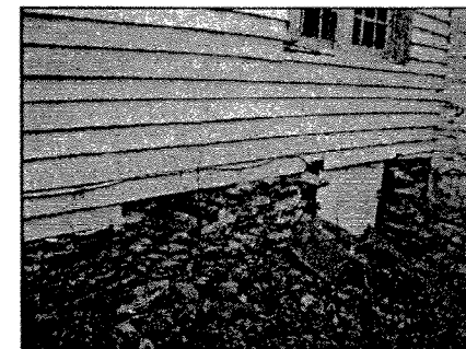
REPAIR AND RESTORE FIELDSTONE FOUNDATION MAINTAINING STRUCTURAL INTEGRITY.
