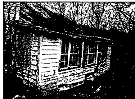
NORTH SHED ADDITION IN DISARRAY, TO BE REMOVED. KITCHEN BEHIND IS ALSO IN DISARRAY WITH PARTS OF THE CEILING HANGING DOWN AND LARGE AMOUNTS OF MOOD DECAY
