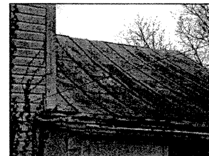
REMOVE OVERGROWTH NORTH SHED ADDITION TO BE REMOVED
