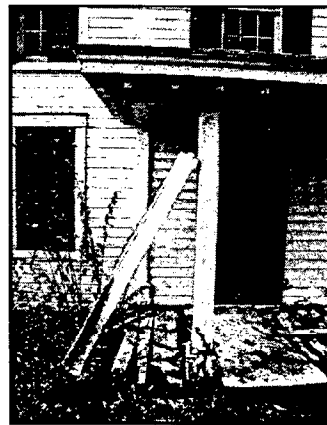
MISSING BRACKET ON CANOPY OVERHANGS, OTHERS STILL IN FAIR CONDITION
