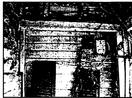
REMOVE EXISTING ROOF MEMBERS AT SOUTH PORCH REMOVE ELECTRICAL WIRING AND FOLIAGE
