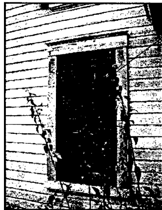
REMOVE EXISTING ROOF MEMBERS AT SOUTH PORCH REMOVE ELECTRICAL WIRING AND FOLIAGE
