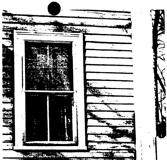
Figure 6. The addition of triple track storm windows, as shown here, greatly improves the thermal performance of existing window assemblies, with a minimal impact on the appearance of the building. (Photo: Baird Smith)
