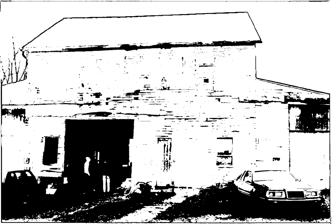
View of mill from east
