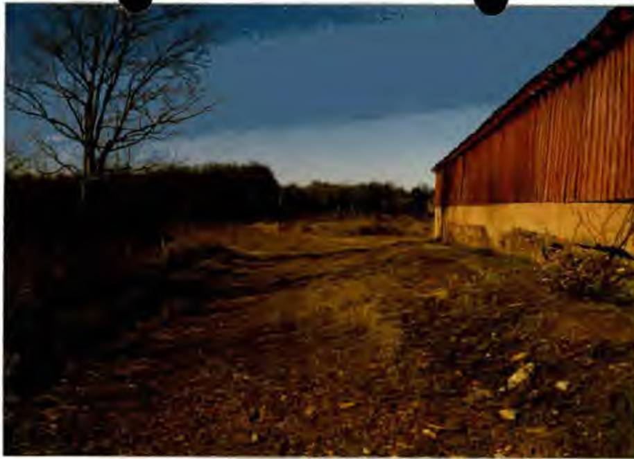
VIEW TOWARD PROPOSED PARKING & ACCESS LANE LOCATED WEST OF RUN-IN SHED
