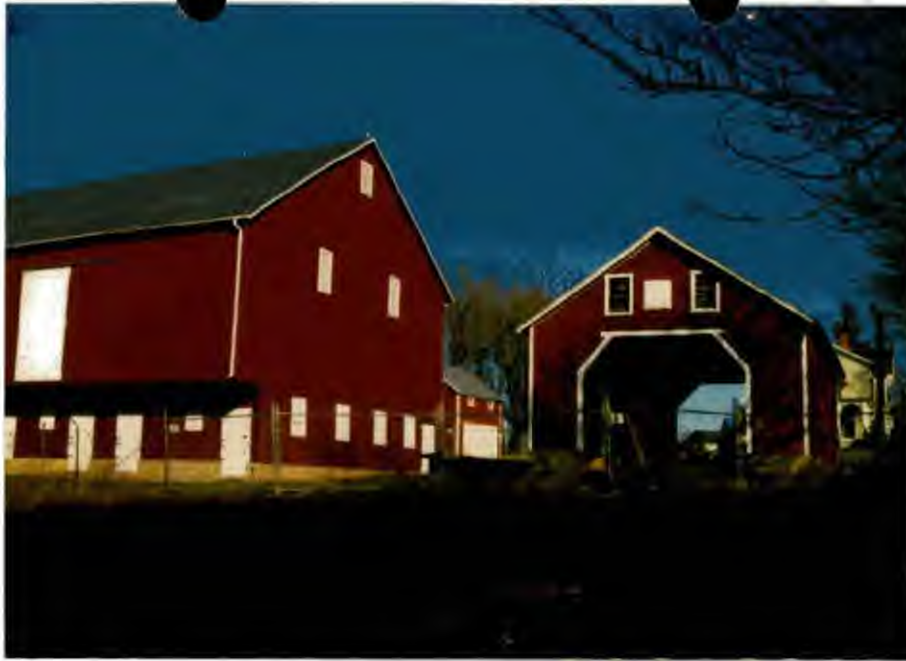
VIEW TOWARD PROPOSED ACCESS LANE & PARKING SOUTH OF BARN.
