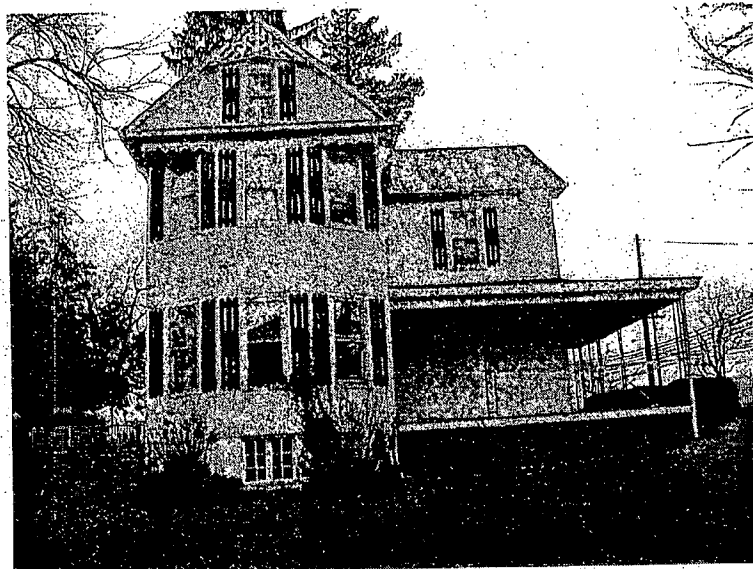
Looking west (temple side)
