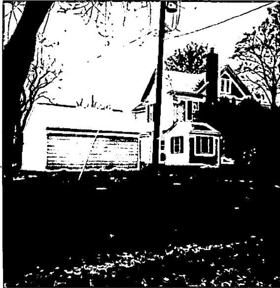
▼ BANKS FARM 3-19-90 ▼ EAST ELEY.- HIST. HOUSE/WELL HOUSE
