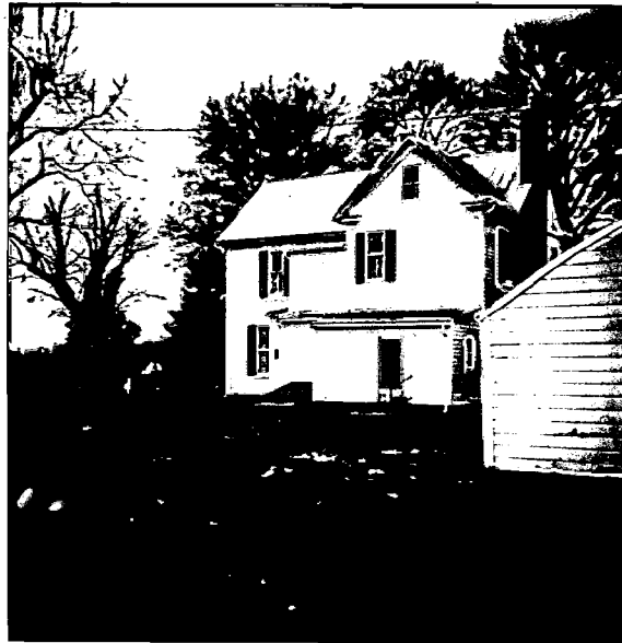
BANKS FARM 3-19-90 WEST ELEV.-HISTORIC HOUSE
