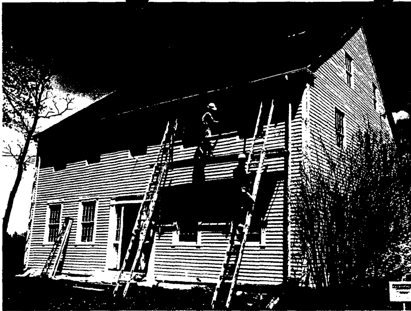
Regular paint maintenance, like spot scraping and painting, has kept this house in good condition for more than 200 years.
