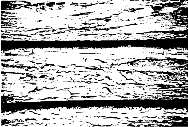
Fig. 9 Cracking, alligatoring, and flaking are evidence of long-term neglect of painted surfaces. The remaining paint on the clapboard shown here can be removed with an electric heat plate and wide-bladed scraper. In addition, unsound wood should be replaced and moisture problems corrected before primer and top coats of paint are applied. Photo: David W. Look, AIA.
