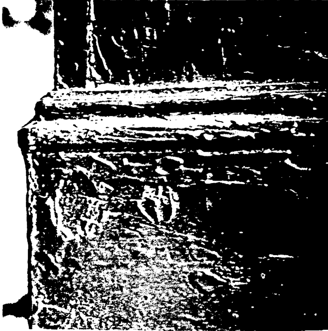
Fig. 10 An excellent example of inadequate scraping before repainting, the problems here are far more than cosmetic. This improperly prepared surface will permit moisture to get behind the paint film which, in turn, will result in chipping and peeling. Photo: Baird M. Smith, AIA.
