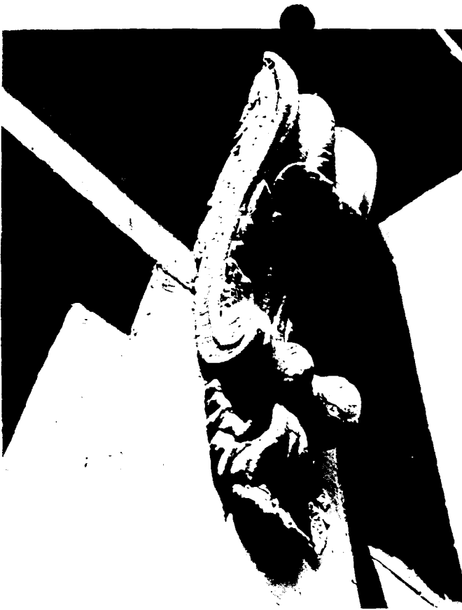
Fig. 1 Excessive paint build-up on architectural details such as this ornamental bracket does not in itself justify total paint removal. If paint is cracked and peeling down to bare wood, however, it should be removed using the gentlest means possible. Photo: David W. Look, AIA.
