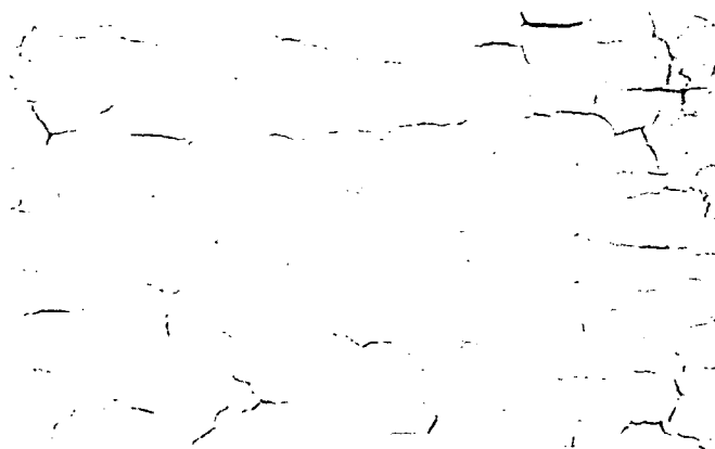
Fig. 5 Crazing—or surface cracking—is an exterior surface condition which can be successfully treated by sanding and painting. Photo: Courtesy, National Decorating Products Association.
