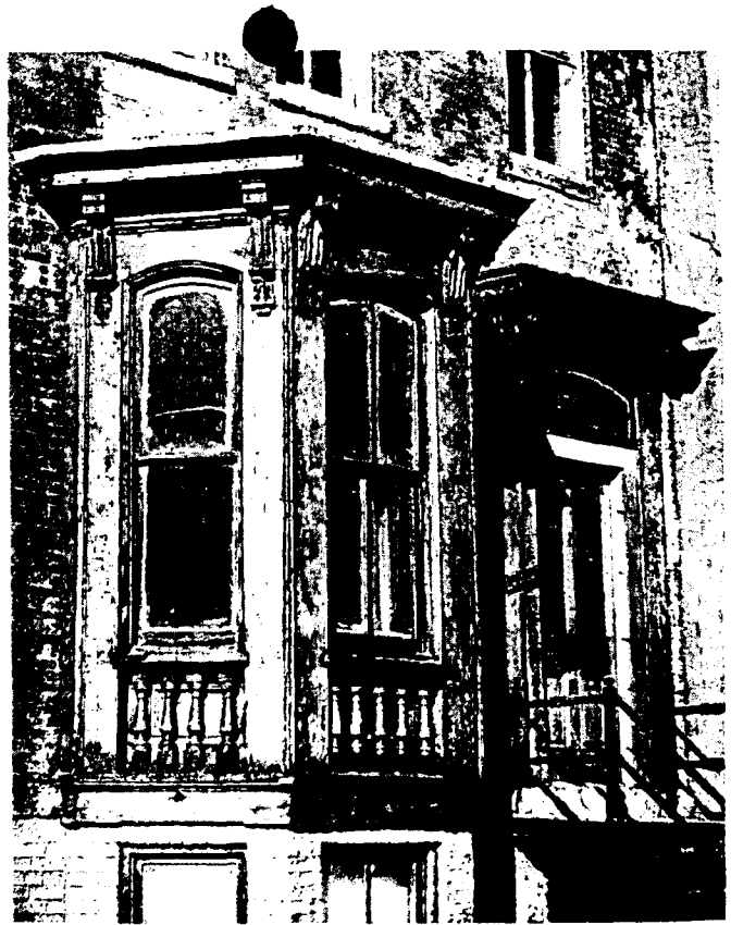
Fig. 2 A traditionally painted bay window has been stripped to bare wood, then varnished. In addition to being historically inaccurate, the varnish will break down faster as a result of the sun's ultraviolet rays than would primer and finish coats of paint. Photo: David W. Look, AIA.
