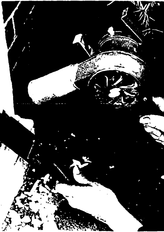
Fig. 14 The nozzle on the electric heat gun permits hot air to be aimed into cavities on solid decorative elements such as this applied column. After the paint has been sufficiently softened, it can be removed with a profiled scraper. Photo: Charles E. Fisher, III.
