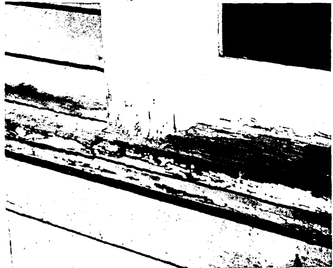
Fig. 4 Paint films wear unevenly depending on exposure and location. Exterior locations which are susceptible to accelerated deterioration are horizontal surfaces such as window sills. These and similar areas will require repainting more often than less vulnerable surfaces. In the case of this window sill where paint has peeled off and adjacent areas have cracked and alligatoring, the paint should be totally removed. Prior to repainting, any weathered wood should be rejuvenated using a solution of 3 cups exterior varnish, 1 oz. paraffin wax, and mineral spirits/paint thinner/or turpentine to make 1 gallon. Liberal brush application should be made. This formula was tested over a 20-year period by the U. S. Department of Agriculture's Forest Products Laboratory and proved to be just as effective as water-repellent preservatives containing pentachlorophenol. After the surface has thoroughly dried (2-3 days of warm weather), the treated surface can be painted. A high quality oil-base primer followed by two top coats of a semi-gloss oil-enamel or latex-enamel paint is recommended. Photo: Baird M. Smith, AIA.
