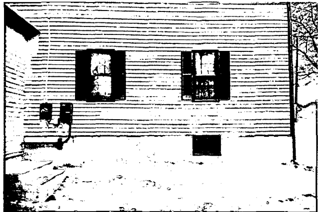
New Landing, Handrail & Steps Replacing window on left
