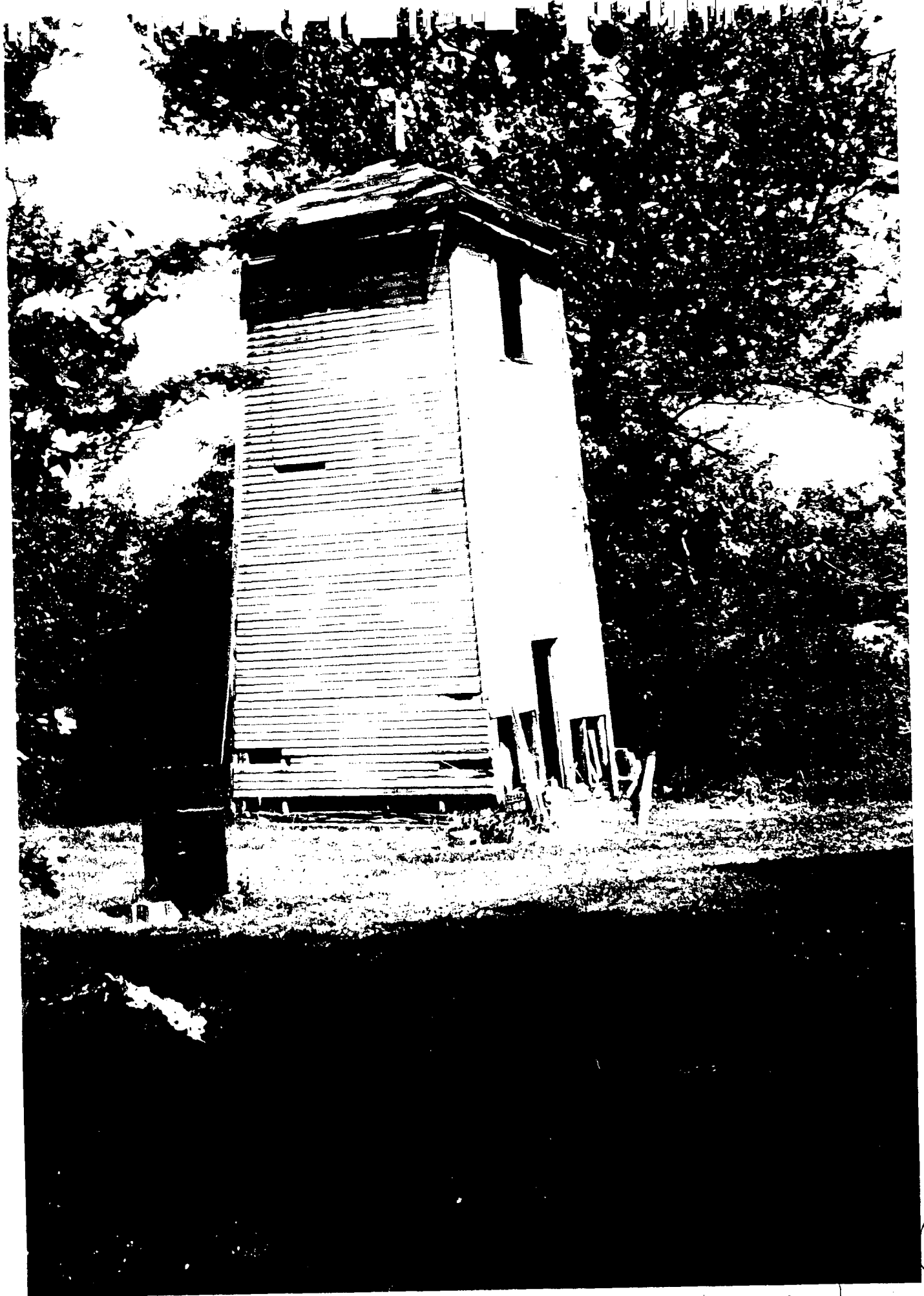
"TOWER HOUSE" 24' x 12' x 16' 2" SUSTAINED FROM PLYWOOD SHEATHING (1941)
