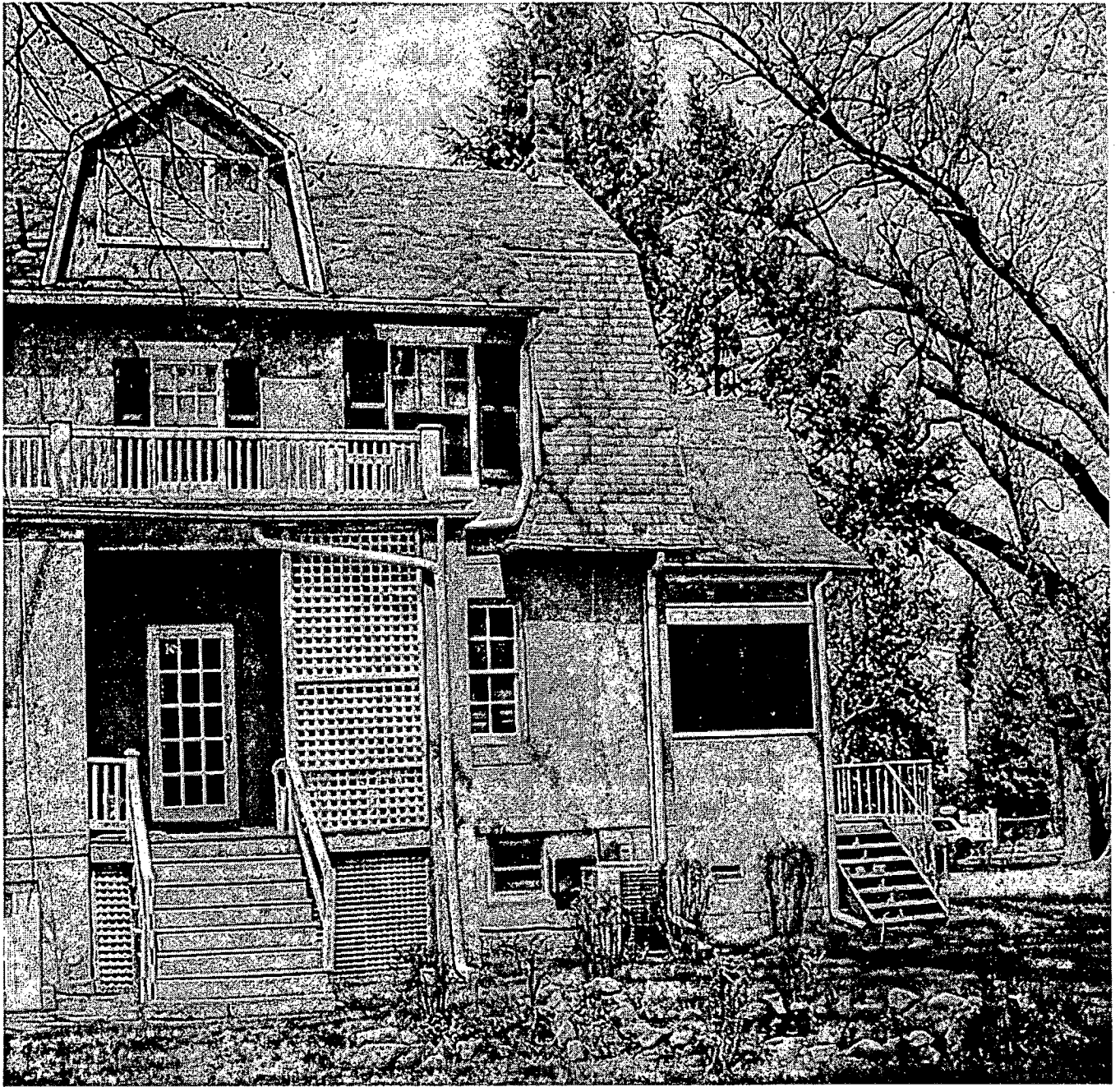
Rear elevation of main block of house
