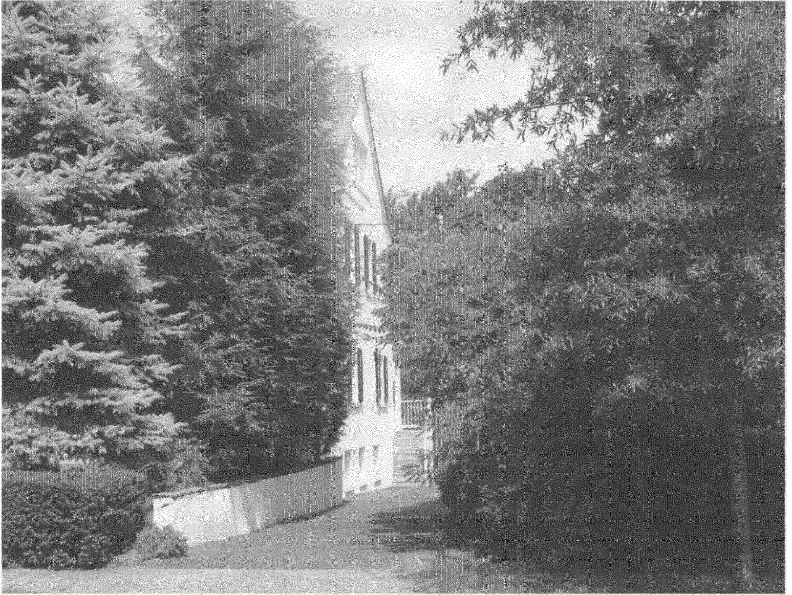
VIEW FROM DRIVEWAY EAST ELEVATION 35 QUINCY STREET
