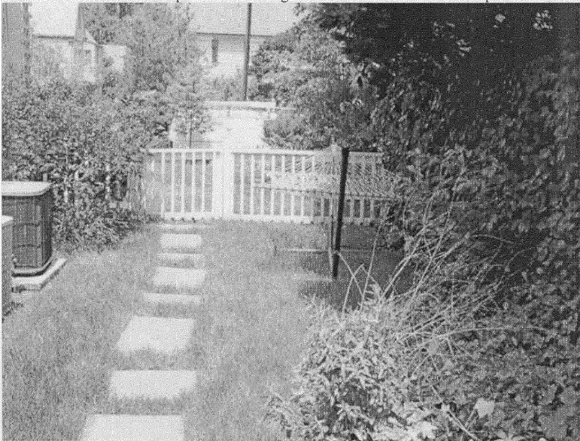
ex. fence to be replaced with 5' high wood fence to meet Code for pool
