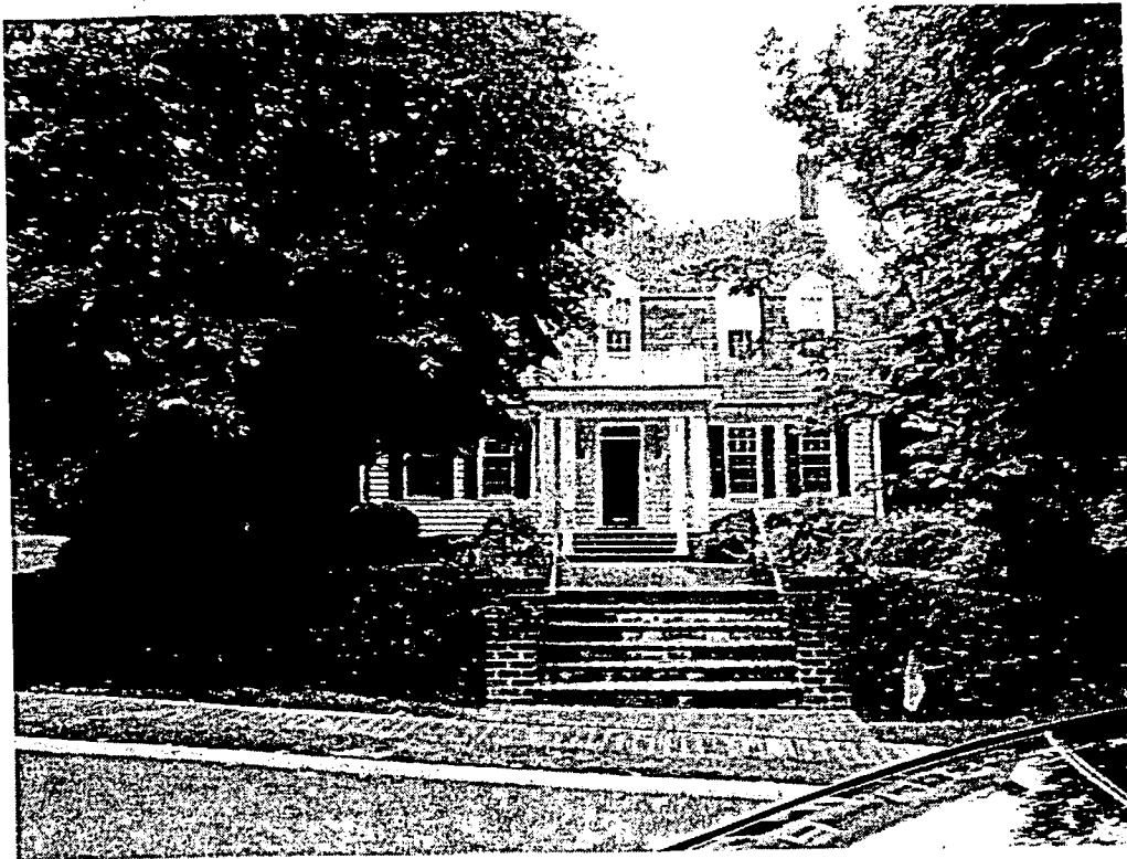
FRONT (NORTH) ELEVATION FROM STREET
