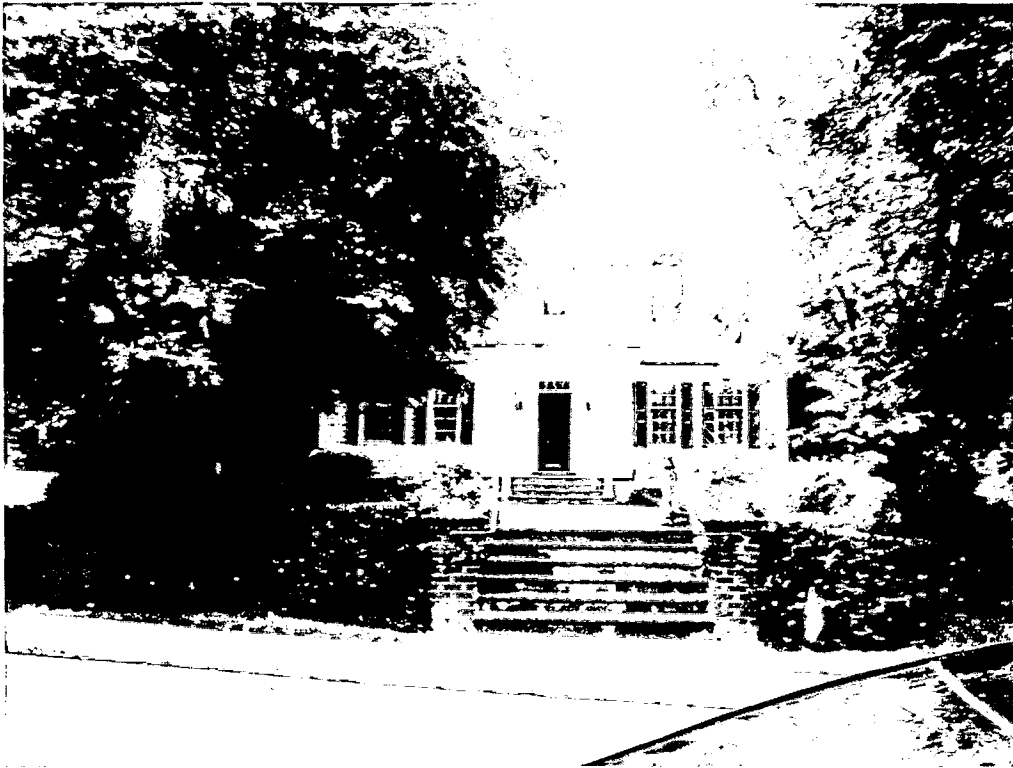
FRONT (NORTH) ELEVATION FROM STREET
