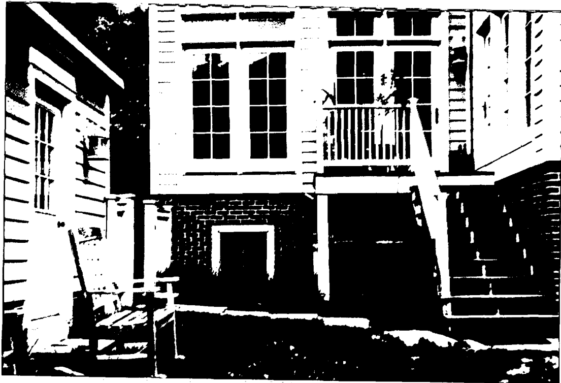
North side, view of Garage and back of house.
