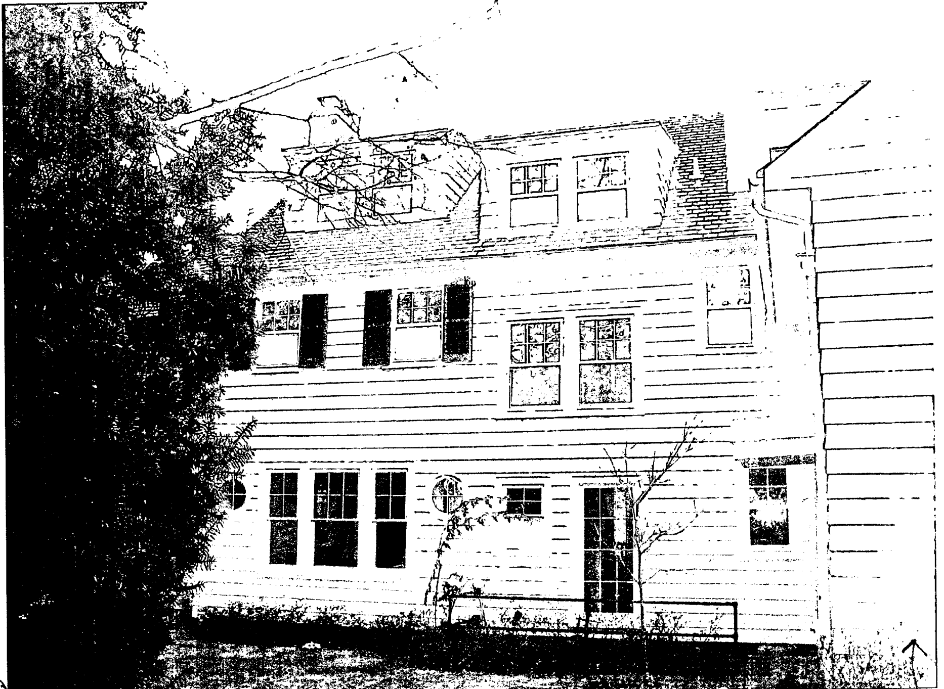
⑥ NORTH ELEVATION, REAR, # 7 MAGNOLIA PARKWAY. 1960 ADDITION IN FOREGROUND # 7/1
