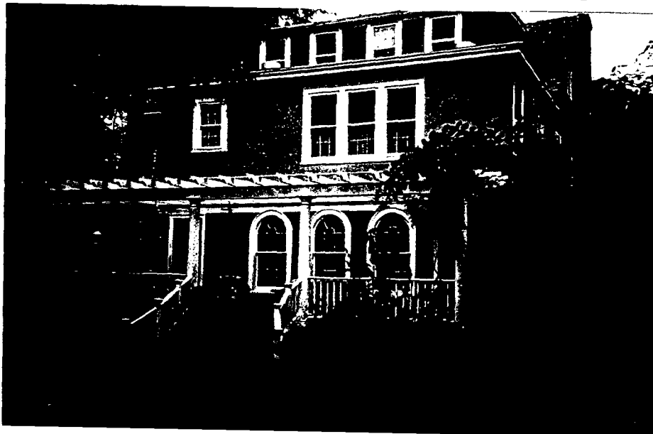
Back (South) facade
