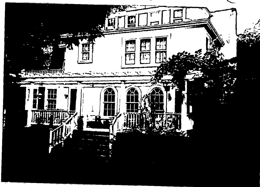
Back (South) facade
