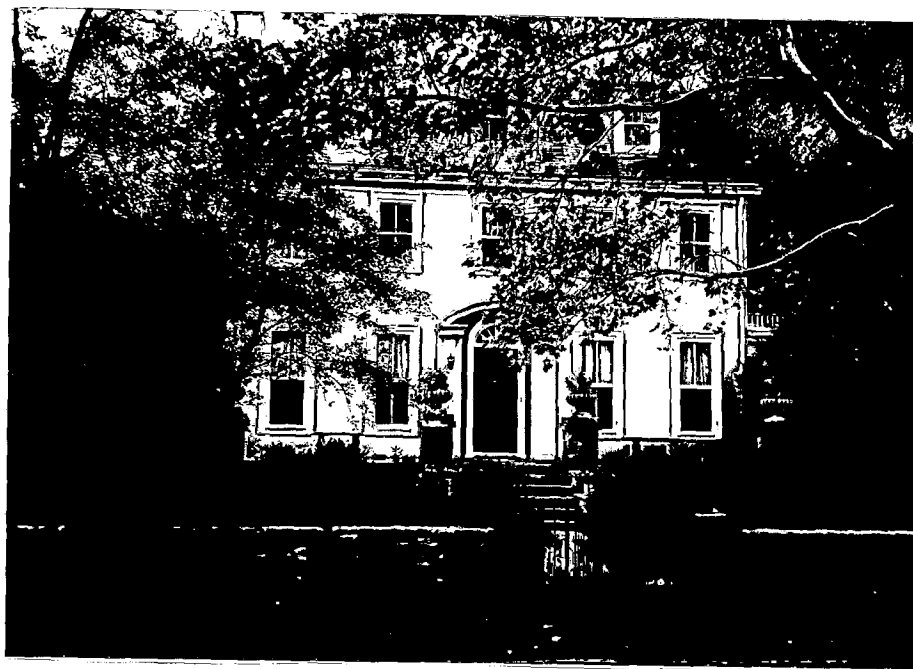
Front (North) facade from street, showing existing door surround
