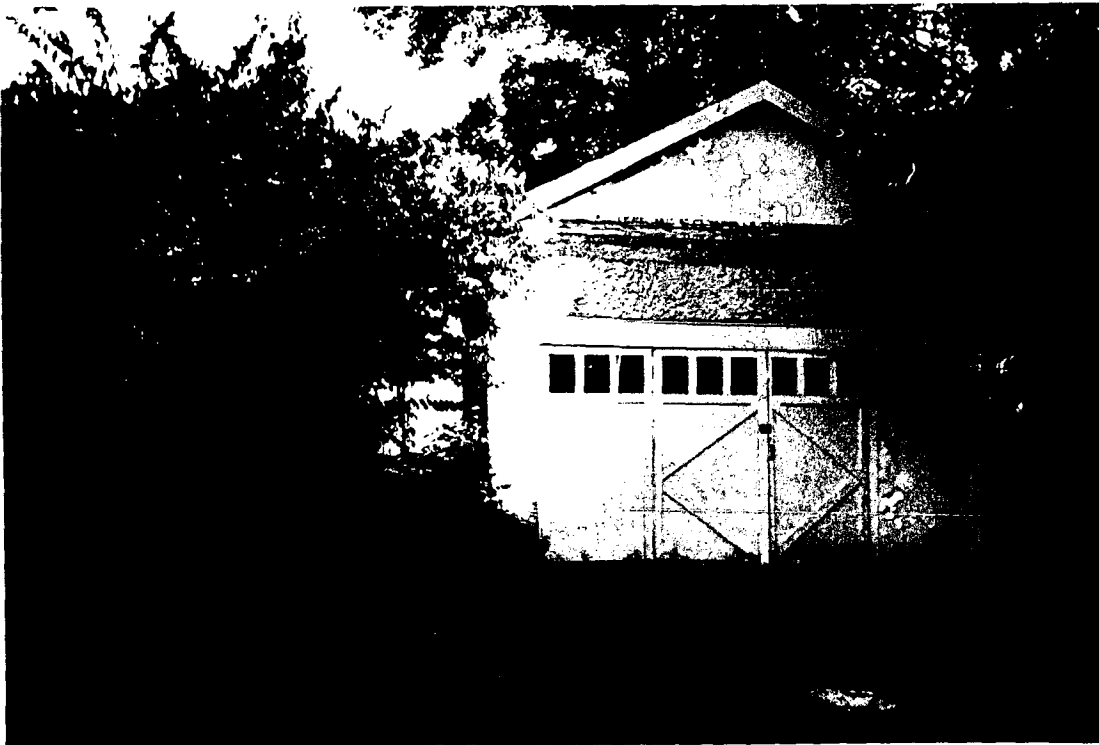
GARAGE, DRIVEWAY & AREA TO BE EXCAVATED FOR ADDITIONAL PARKING
