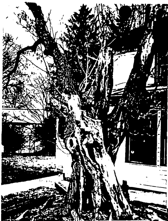
Tree on side of house is completely rotted away. ①
