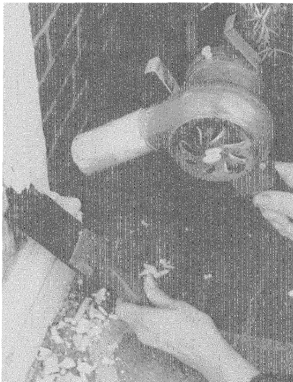
Fig. 14 The nozzle on the electric heat gun permits hot air to be aimed into cavities on solid decorative elements such as this applied column. After the paint has been sufficiently softened, it can be removed with a profiled scraper. Photo: Charles E. Fisher, III.
