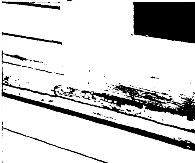
Fig. 4 Paint films wear unevenly depending on exposure and location. Exterior locations which are susceptible to accelerated deterioration are horizontal surfaces such as window sills. These and similar areas will require repainting more often than less vulnerable surfaces. In the case of this window sill where paint has peeled off and adjacent areas have cracked and alligatored, the paint should be totally removed. Prior to repainting, any weathered wood should be rejuvenated using a solution of 3 cups exterior varnish, 1 oz. paraffin wax, and mineral spirits/paint thinner/or turpentine to make 1 gallon. Liberal brush application should be made. This formula was tested over a 20-year period by th. U.S. Department of Agriculture's Forest Products Laboratory and proved to be just as effective as water-repellent preservatives containing pentachlorophenol. After the surface has thoroughly dried (2-3 days of warm weather), the treated surface can be painted. A high quality oil-base primer followed by two top coats of a semi-gloss oil-enamel or latex-enamel paint is recommended. Photo: Baird M. Smith, AIA.
