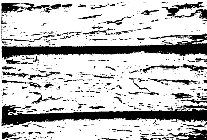
Fig. 9 Cracking, alligatoring, and flaking are evidence of long-term neglect of painted surfaces. The remaining paint on the clapboard shown here can be removed with an electric heat plate and wide-bladed scraper. In addition, unsound wood should be replaced and moisture problems corrected before primer and top coats of paint are applied. Photo: David W. Look, AIA.
