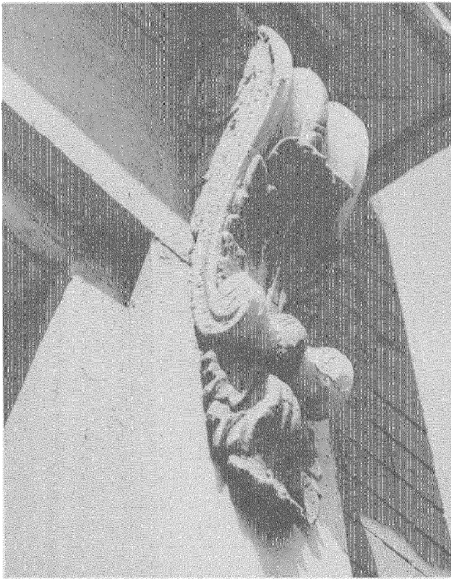
Fig. 1 Excessive paint build-up on architectural details such as this ornamental bracket does not in itself justify total paint removal. If paint is cracked and peeling down to bare wood, however, it should be removed using the gentlest means possible. Photo: David W. Look, AIA.
