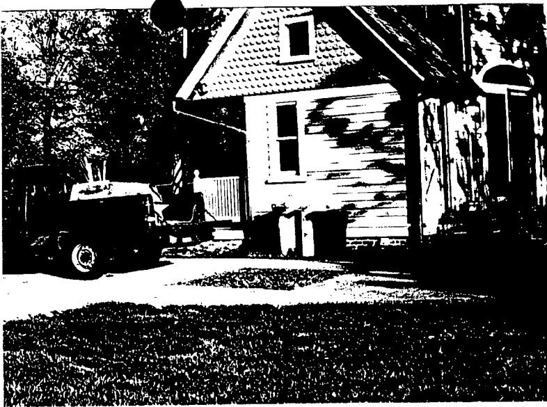
① North facade of resource (rear) Showing PPO near entryway addition
