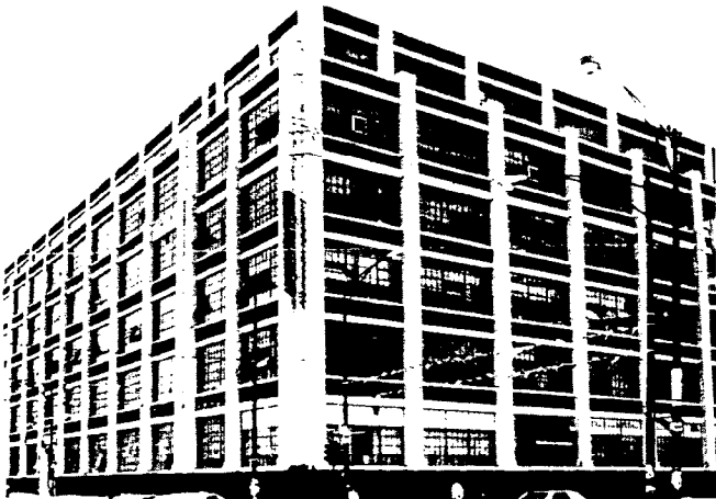
Fig. 10 a. A six-story concrete manufacturing building prior to the replacement of the steel pivot windows. Photo: Charles Parrott.
