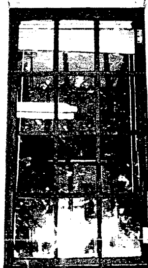
Fig. 6 f. View from the outside of the completely refurbished window. In addition to the steel repair and the installation of vinyl weatherstripping, the exterior was caulked with polyurethane and the single glass was replaced with individual lights of thermal glass. The repaired and upgraded windows have comparable energy efficiency ratings to new replacement units while retaining the historic steel sash, frames and subframes.
