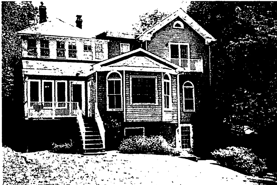
VIEW OF WEST/REAR FACADE FROM BACKYARD 1970'S ONE-STORY ADDITIONS PROPOSED TO BE REMOVED
