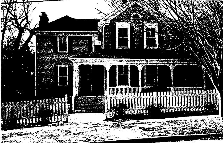
VIEW OF EAST/STREET FACADE FROM WARWICK PLACE
