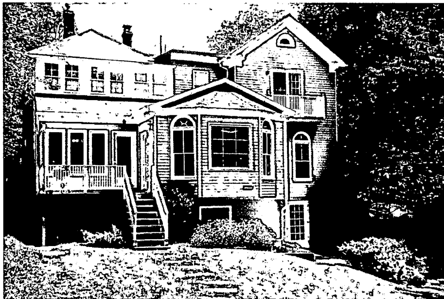
VIEW OF WEST/REAR FACADE FROM BACKYARD 1970'S ONE-STORY ADDITIONS PROPOSED TO BE REMOVED
