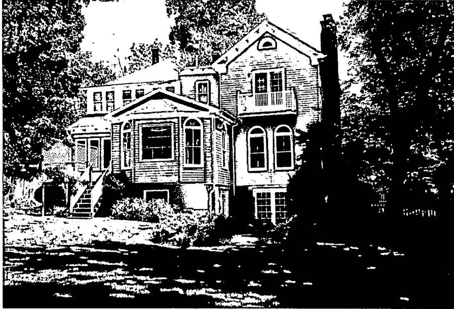
VIEW OF WEST/REAR FACADE FROM BACKYARD 1970'S ONE-STORY ADDITIONS PROPOSED TO BE REMOVED
