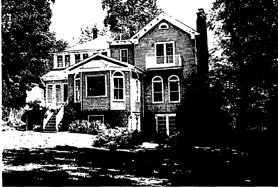
VIEW OF WEST/REAR FACADE FROM BACKYARD 1970'S ONE-STORY ADDITIONS PROPOSED TO BE REMOVED
