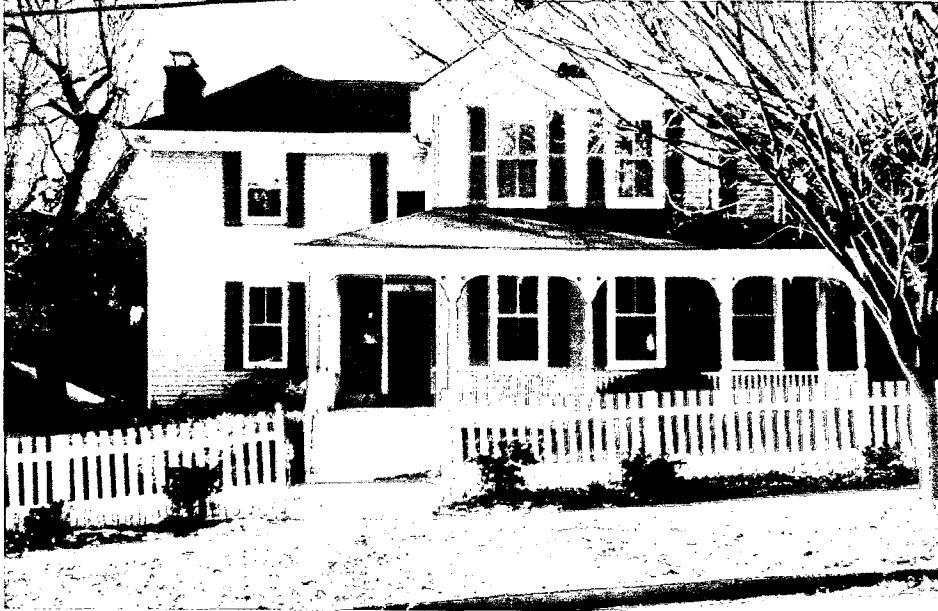
VIEW OF EAST/STREET FACADE FROM WARWICK PLACE
