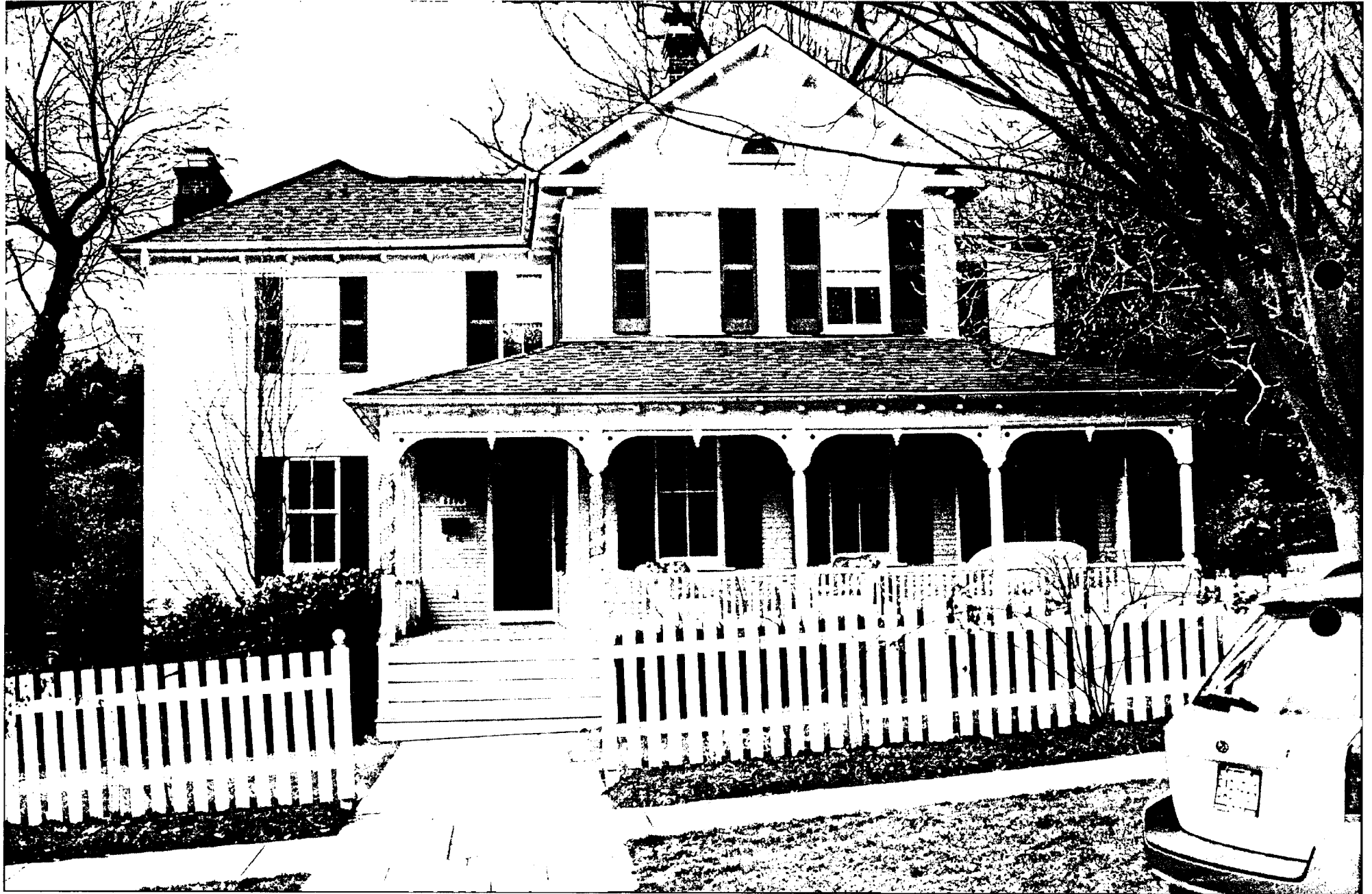
⑤ 5806 WARWICK PLACE (ADJACENT SOUTH PROPERTY)
