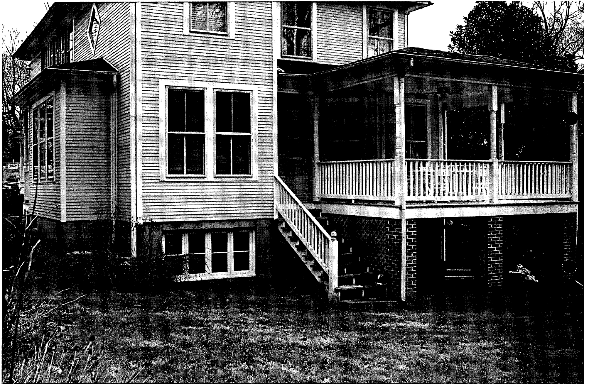
Ⓝ OBLIQUE VIEW OF NORTHWEST CORNER (1980'S STAIR @ NORTH SIDE + 1990'S PORCH)
