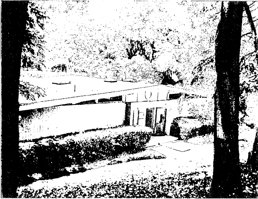
1. Eastern elevation of existing bathhouse to be replaced
