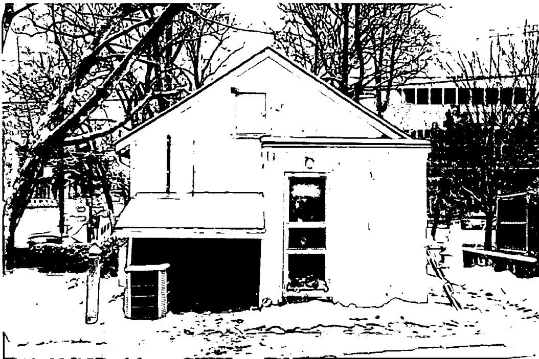
Before renovation, view from the West.
