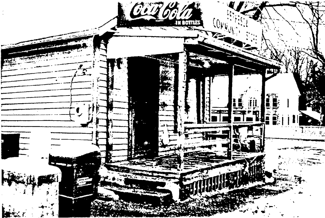
Bethesda Community Store, 8804 Old Georgetown Road, Bethesda, Maryland: Before renovation, view from East.
