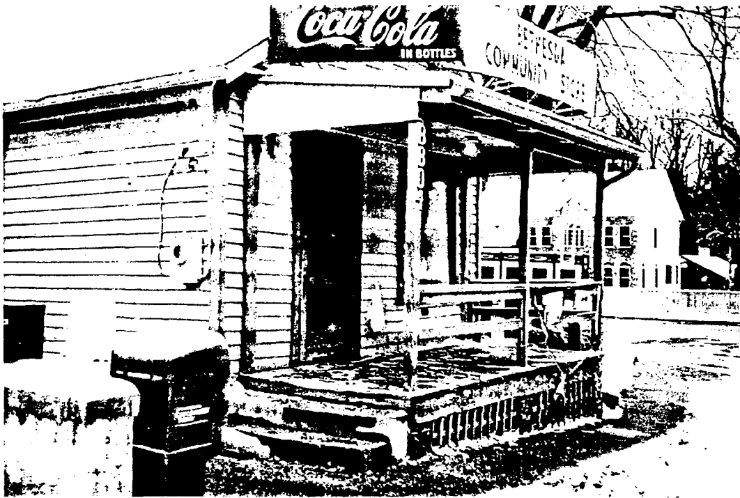
Bethesda Community Store, 8804 Old Georgetown Road, Bethesda, Maryland: Before renovation, view from East.
