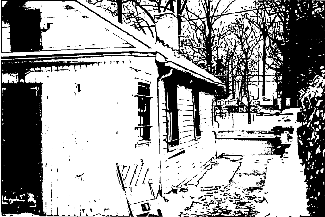
Bethesda Community Store, 8804 Old Georgetown Road, Bethesda, Maryland: Before renovation, view from Southwest.
