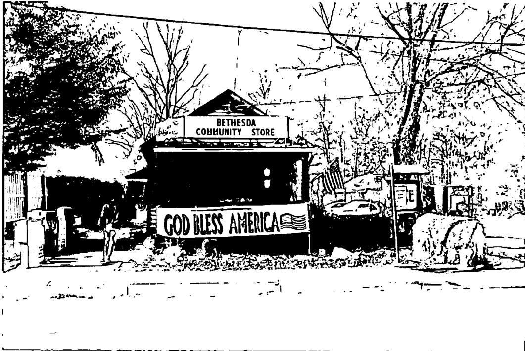
Bethesda Community Store, 8804 Old Georgetown Road, Bethesda, Maryland: After renovation, view from East.
