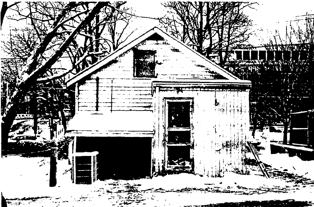
Before renovation, view from the West.
