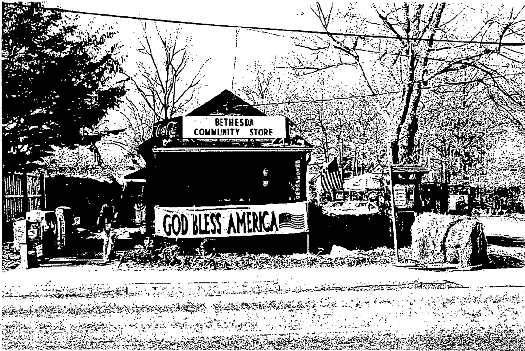
Bethesda Community Store, 8804 Old Georgetown Road, Bethesda, Maryland: After renovation, view from East.
