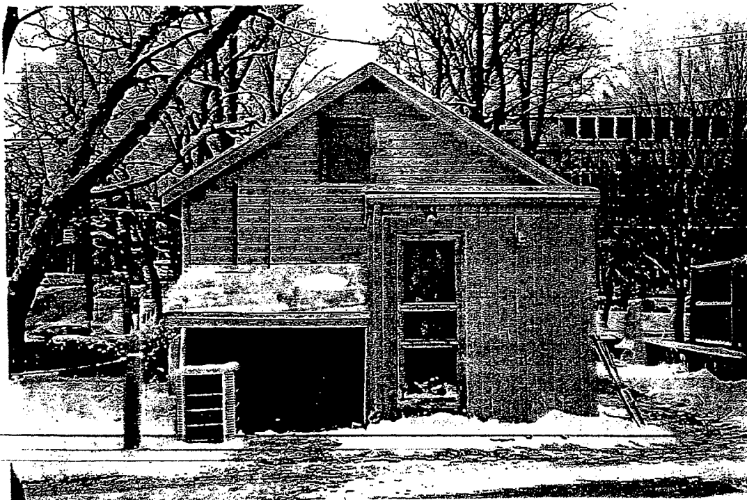
Before renovation, view from the West.
