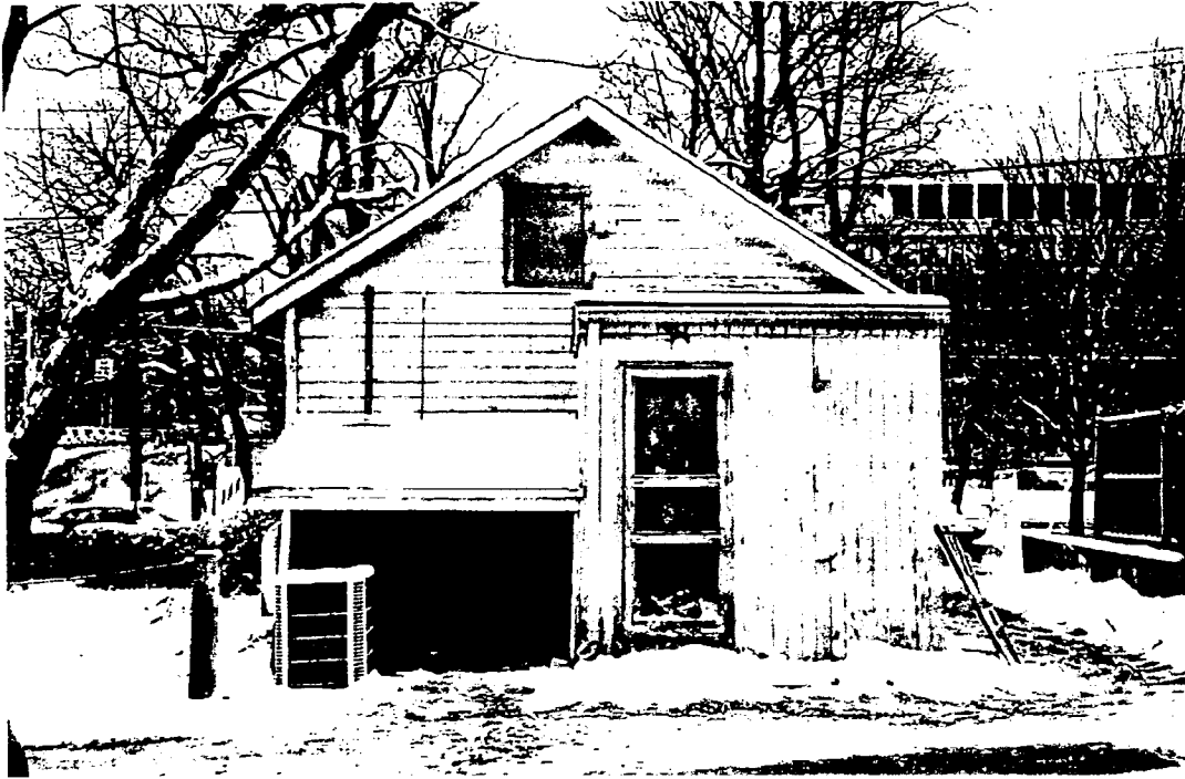
Before renovation, view from the West.
