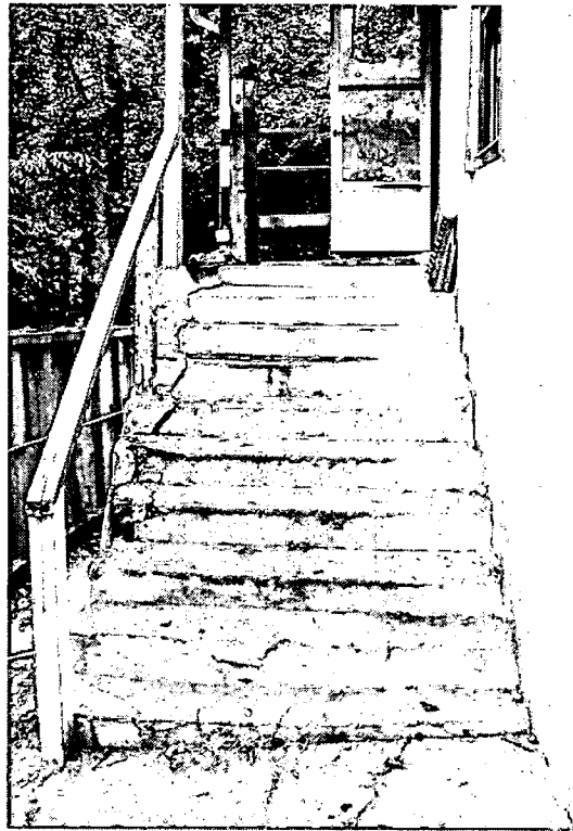
South Elevation Steps, deteriorated
