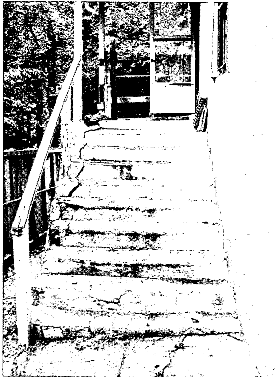
South Elevation Steps, deteriorated
