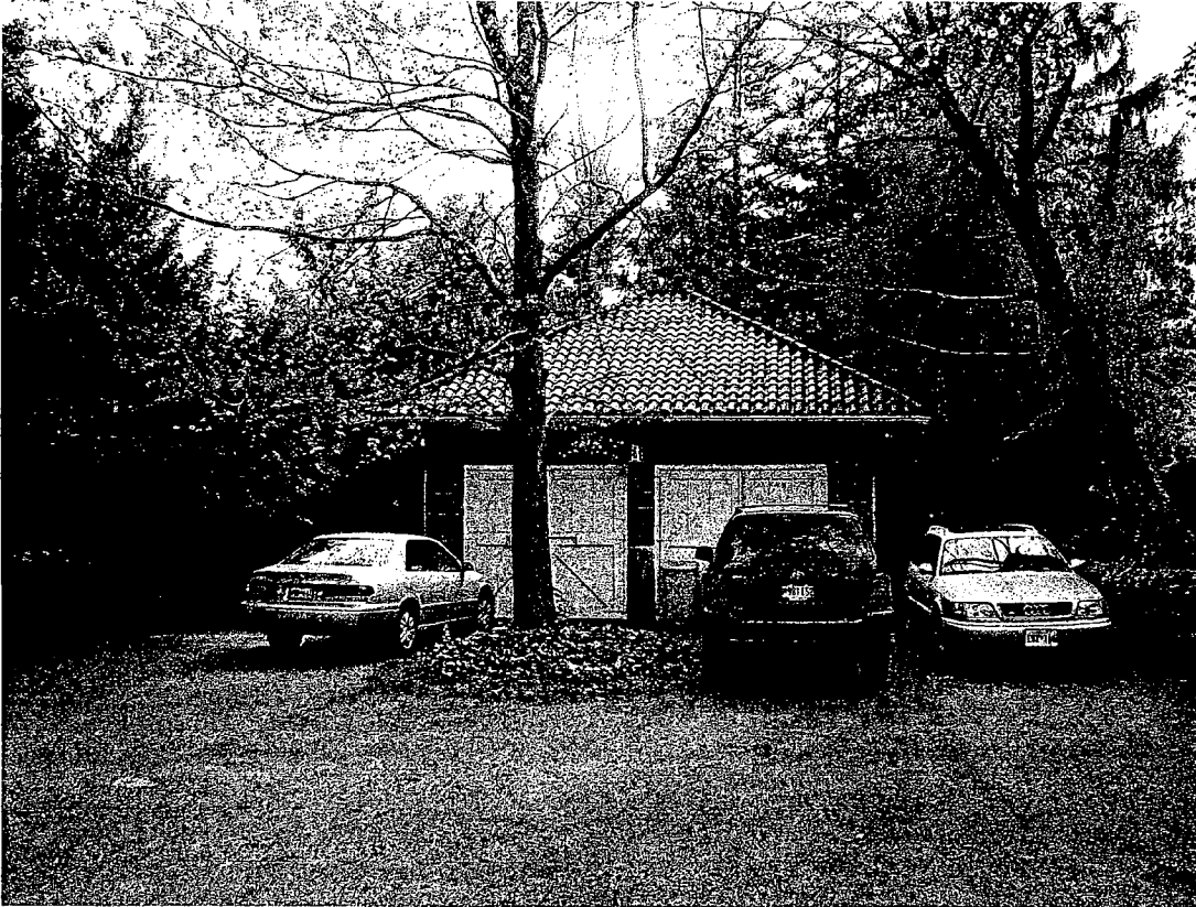
EXISTING GARAGE ON PROPERTY
