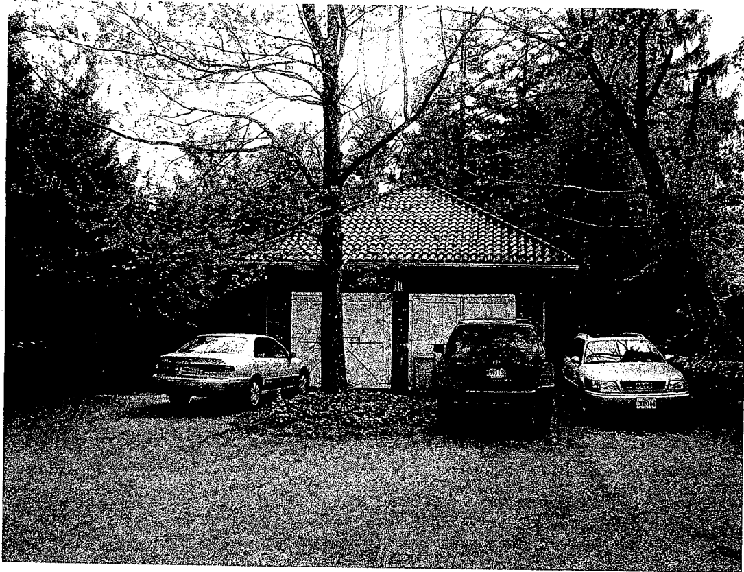
EXISTING GARAGE ON PROPERTY
