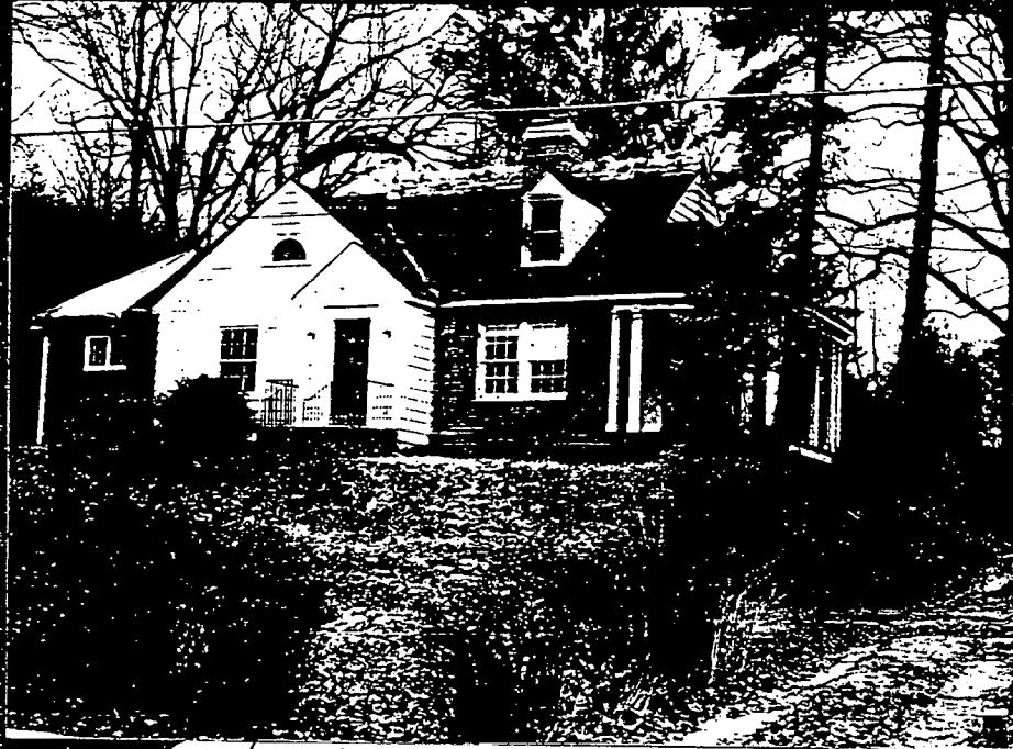
West Elevation View from direction of Durrey Street
