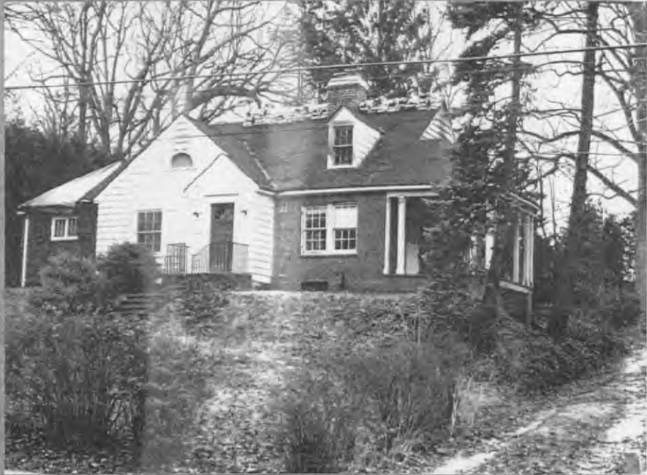
West Elevation View from direction of Surrey Street.
