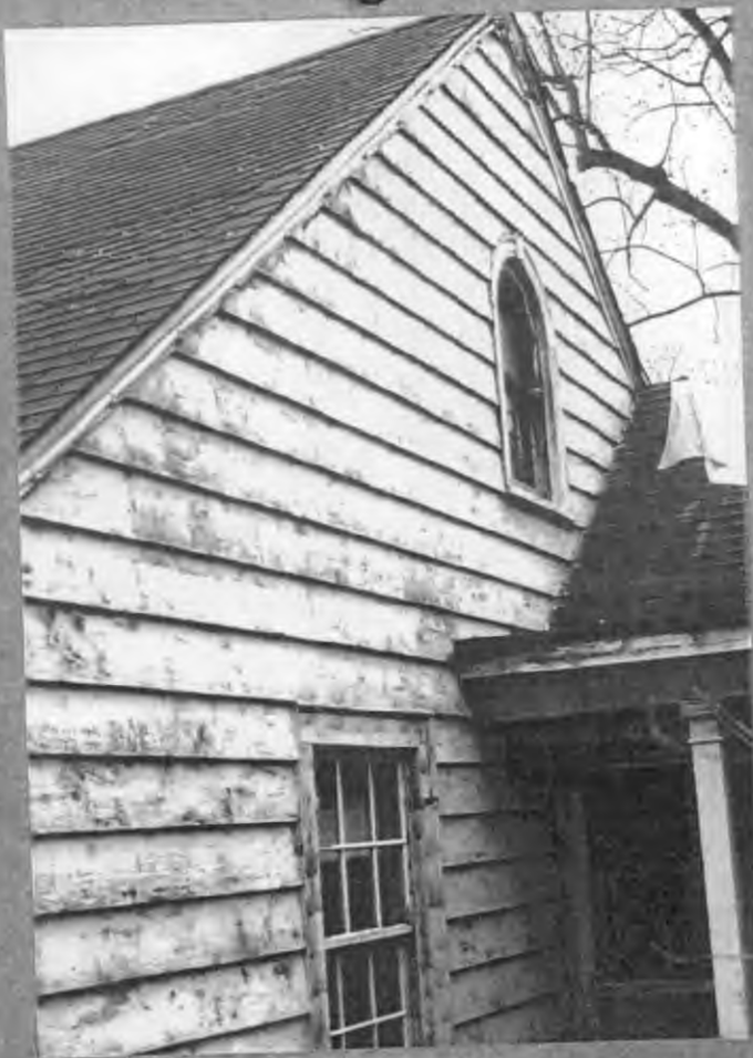
North Elevation Gable
