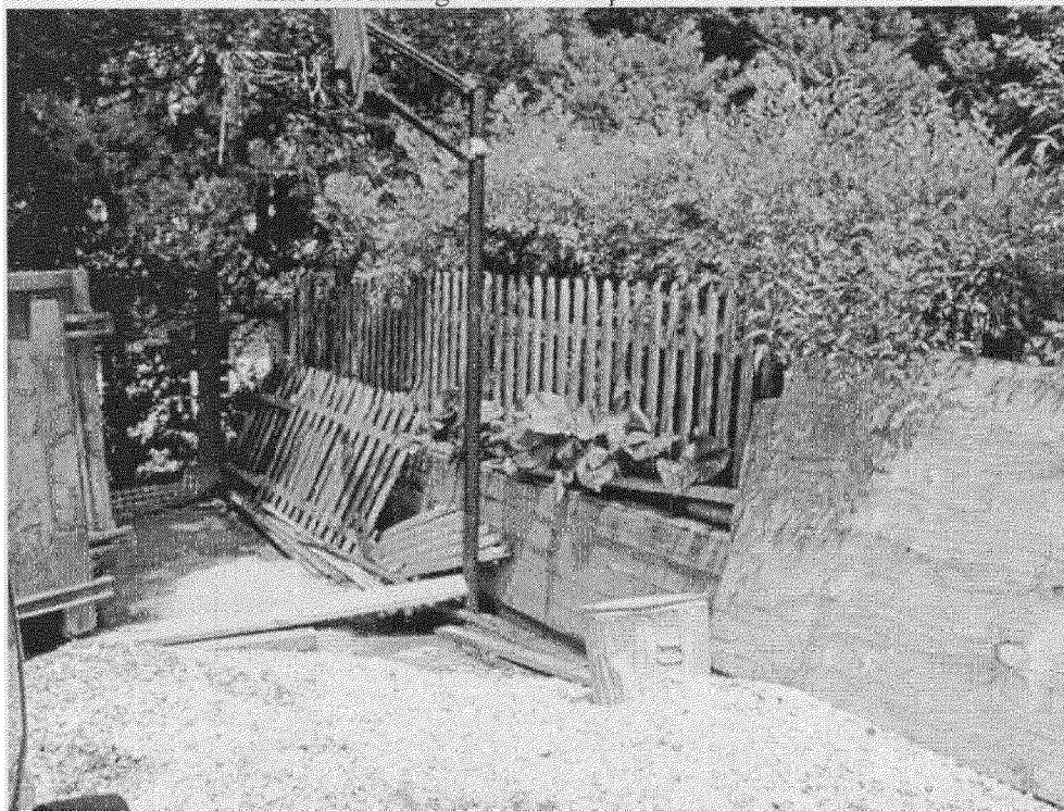
timber retaining wall to be replaced with stone
