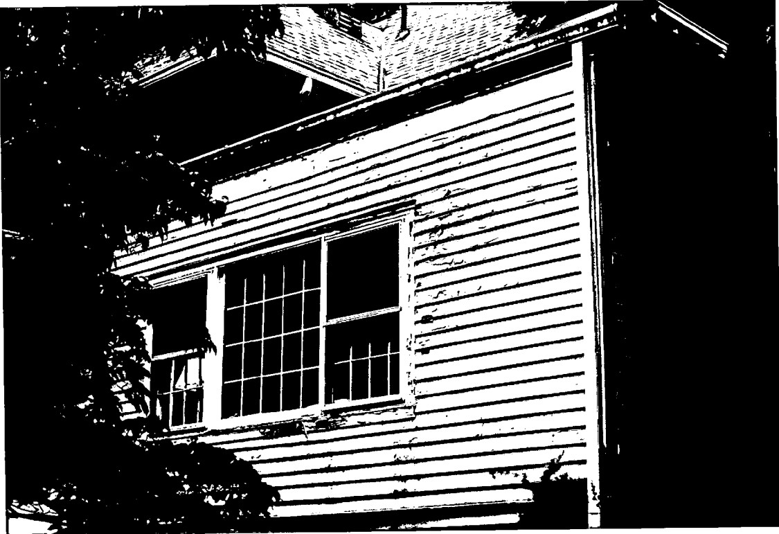
NORTH FACADE showing water damage
