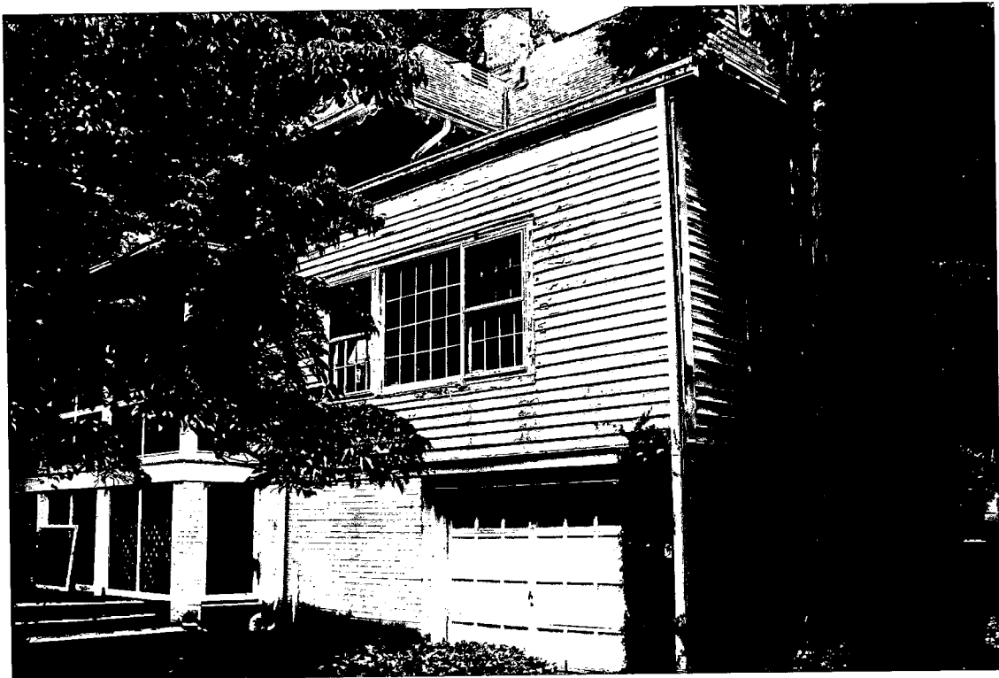
NORTH FACADE looking from northwest
