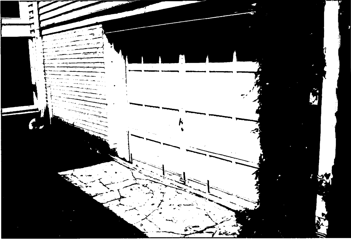
CLOSEUP OF NORTH FACADE looking from northwest
