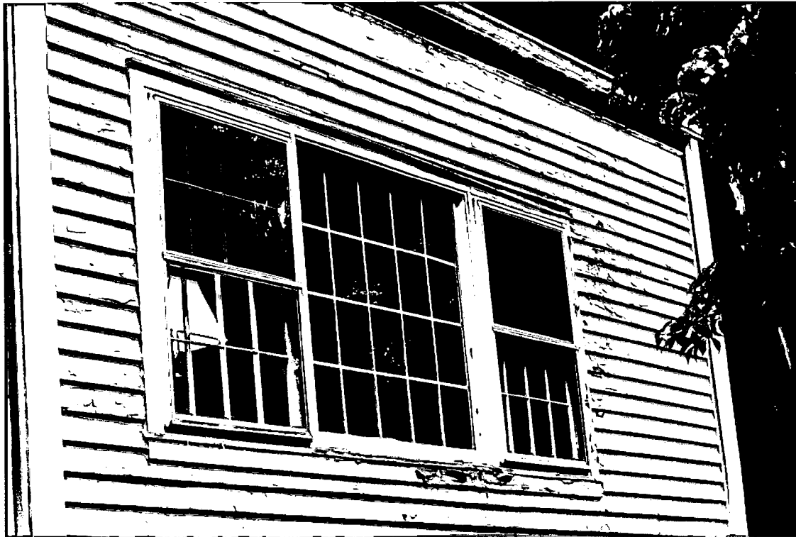
CLOSEUP OF NORTH FACADE looking from northeast
