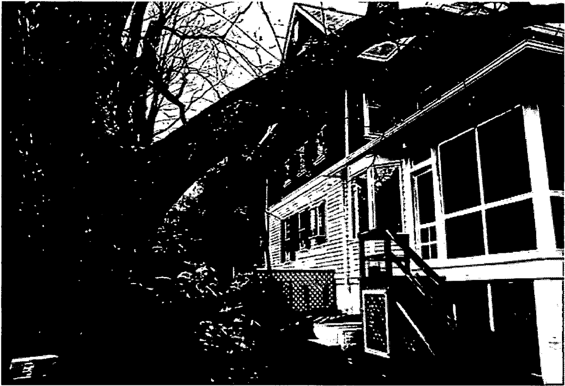
4923 Dorset Avenue, Somerset Historic District East elevation.
