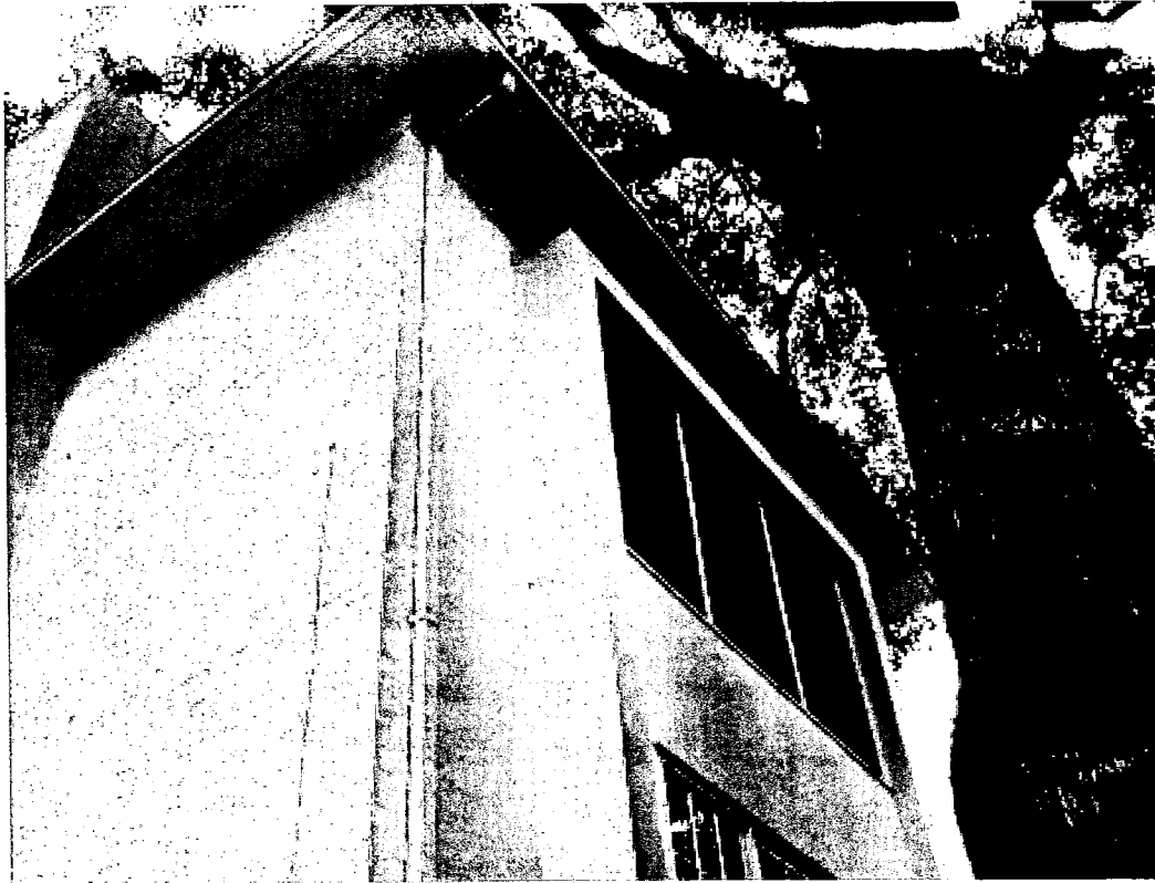
REAR VIEW OF EXISTING BOX BAY TO BE REMOVED AND REPLACED WITH BOW WINDOWS AND PANELS
