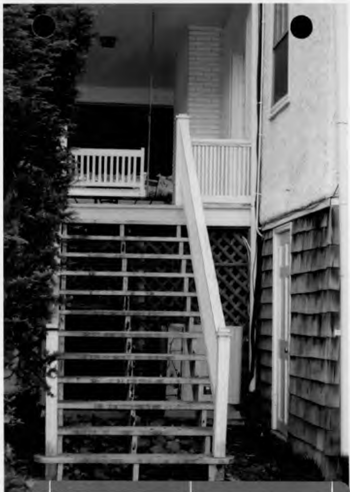
Existing Side Porch Steps
