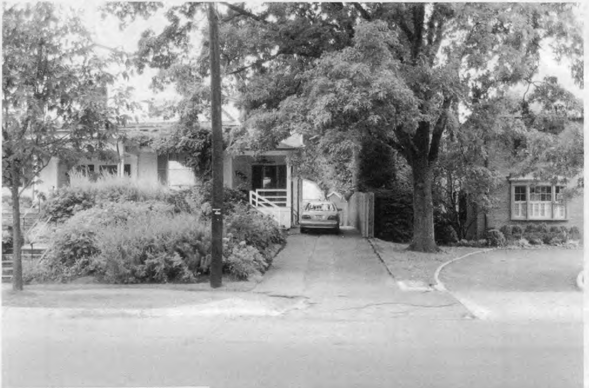
19 Grafton Street, Chevy Chase View Looking North proposed new Apron, Sidewalk and driveway
