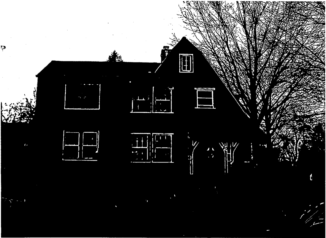
FRONT View From Hesketh Street ↑
