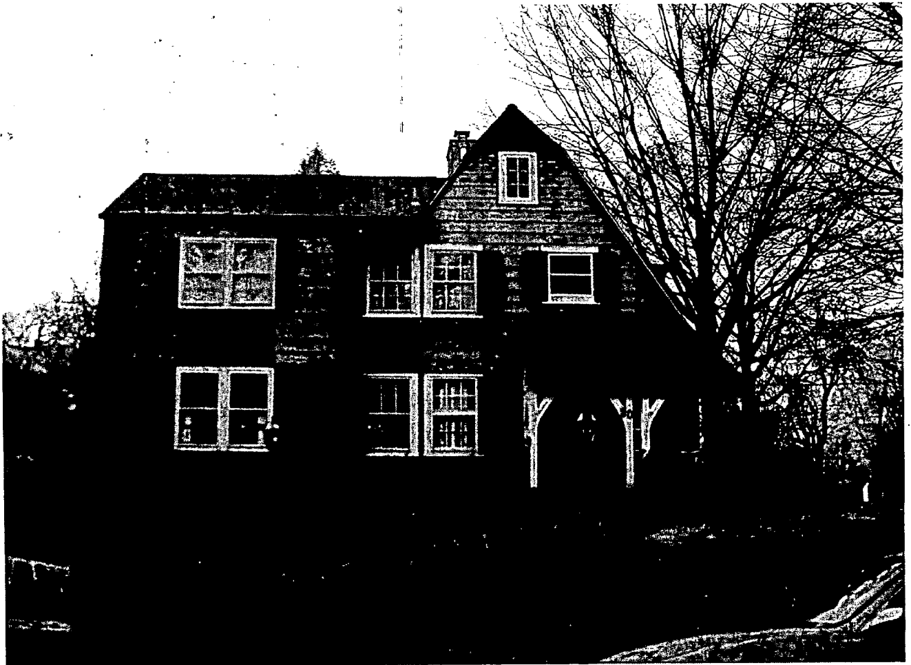
Front View From Hesketh Street ↑
