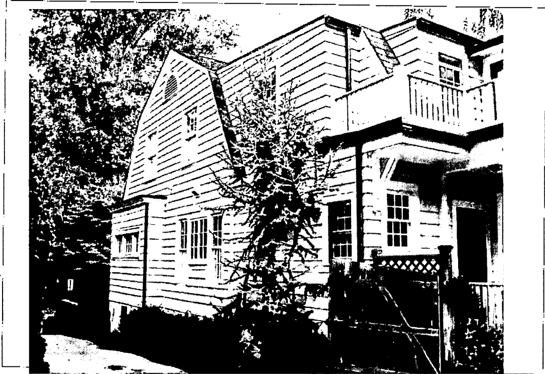
Detail: View of SW Corner
