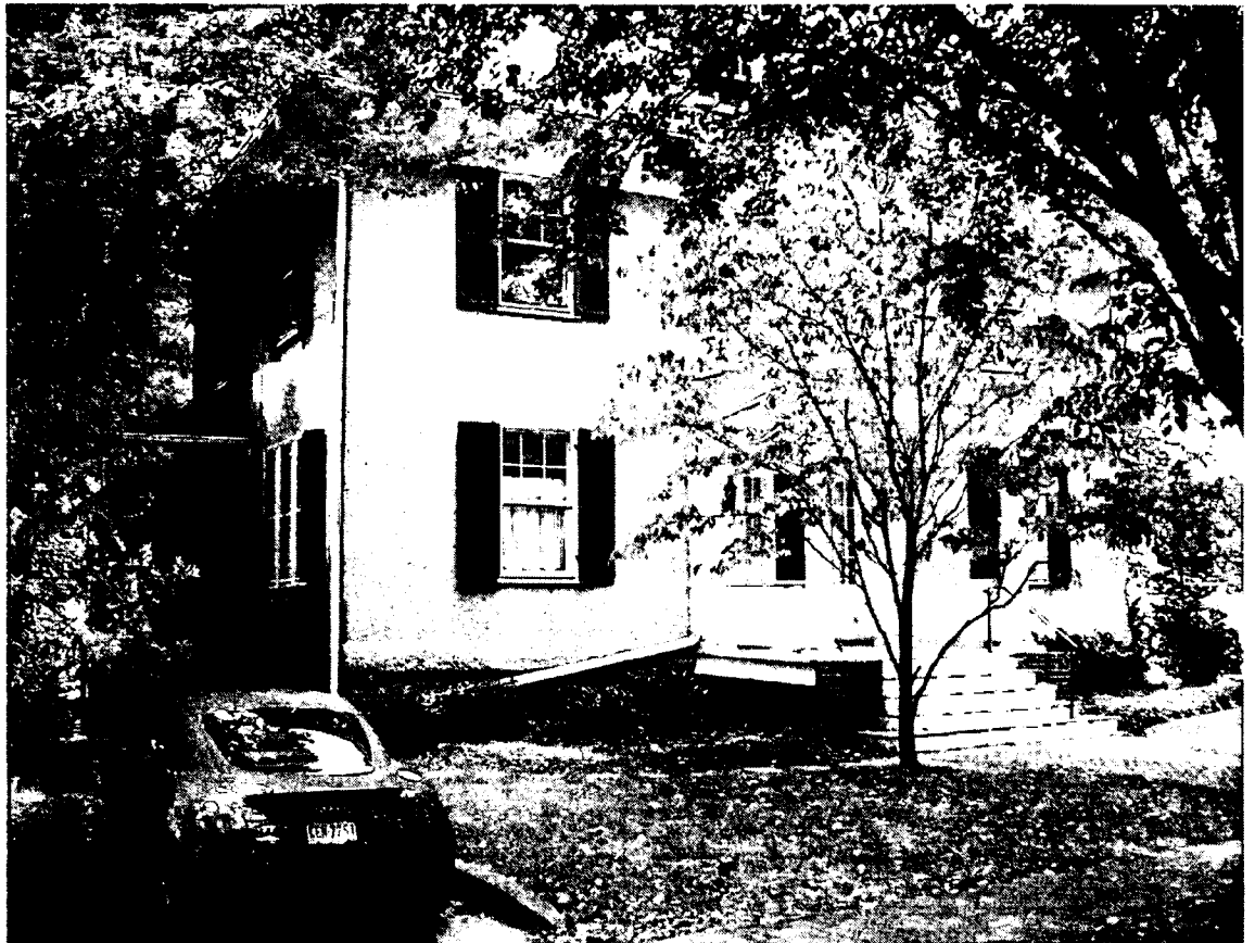
North and East side from Irving Street
