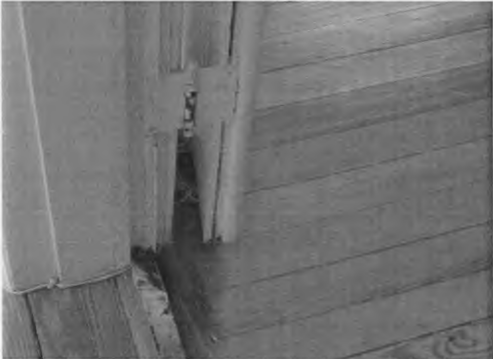
Interior/Former Exterior door in master bedroom(detail)
