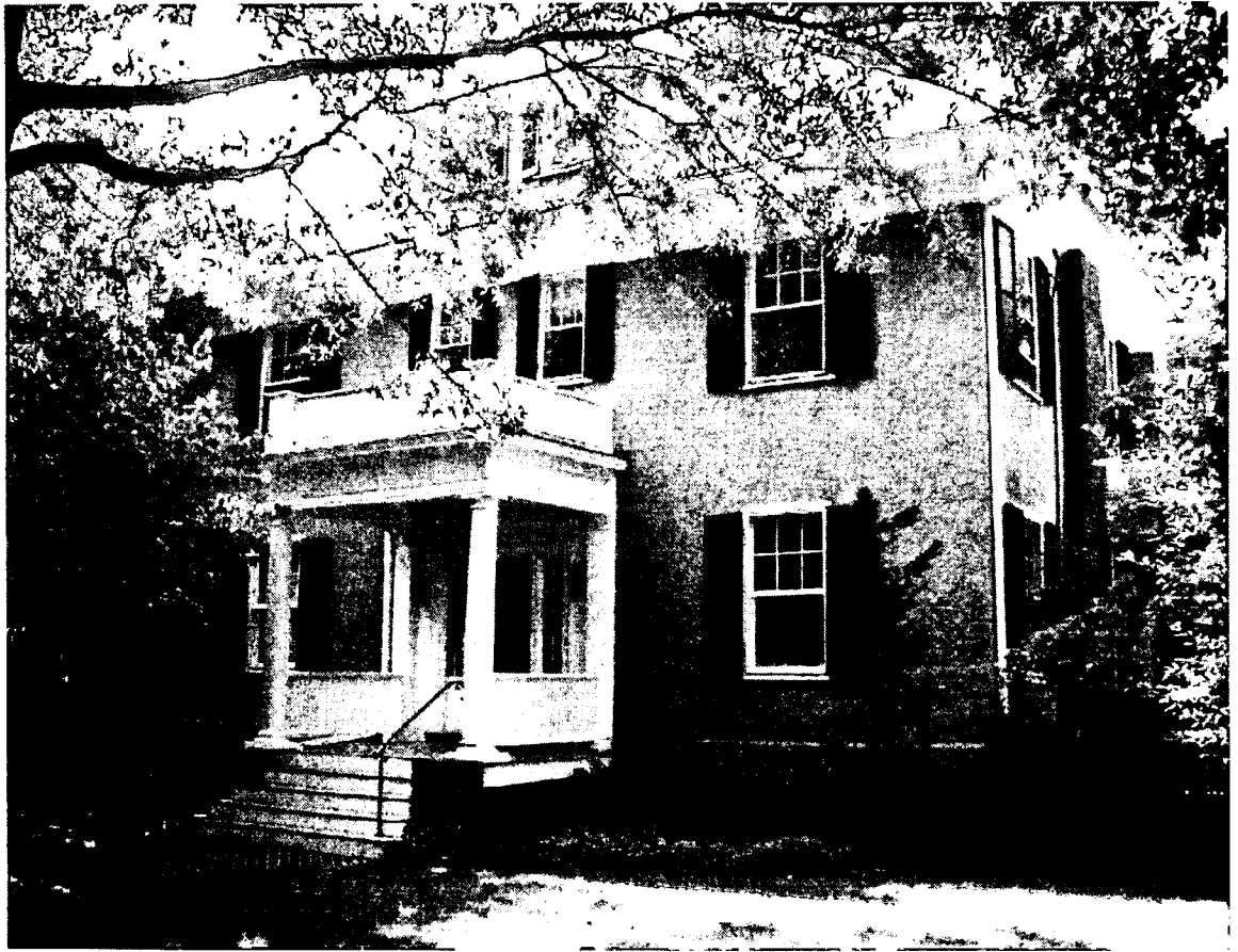
North and West side from Irving Street
