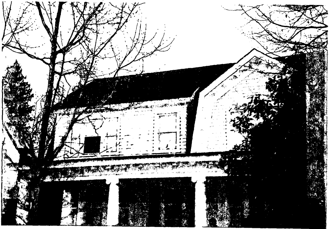
6 Hesketh Street (Above) w/ asphalt roof
