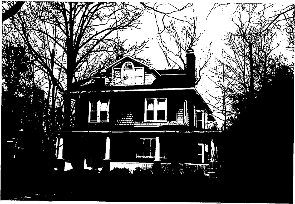
3 Hesketh Street (Above) w/ asphalt roof
