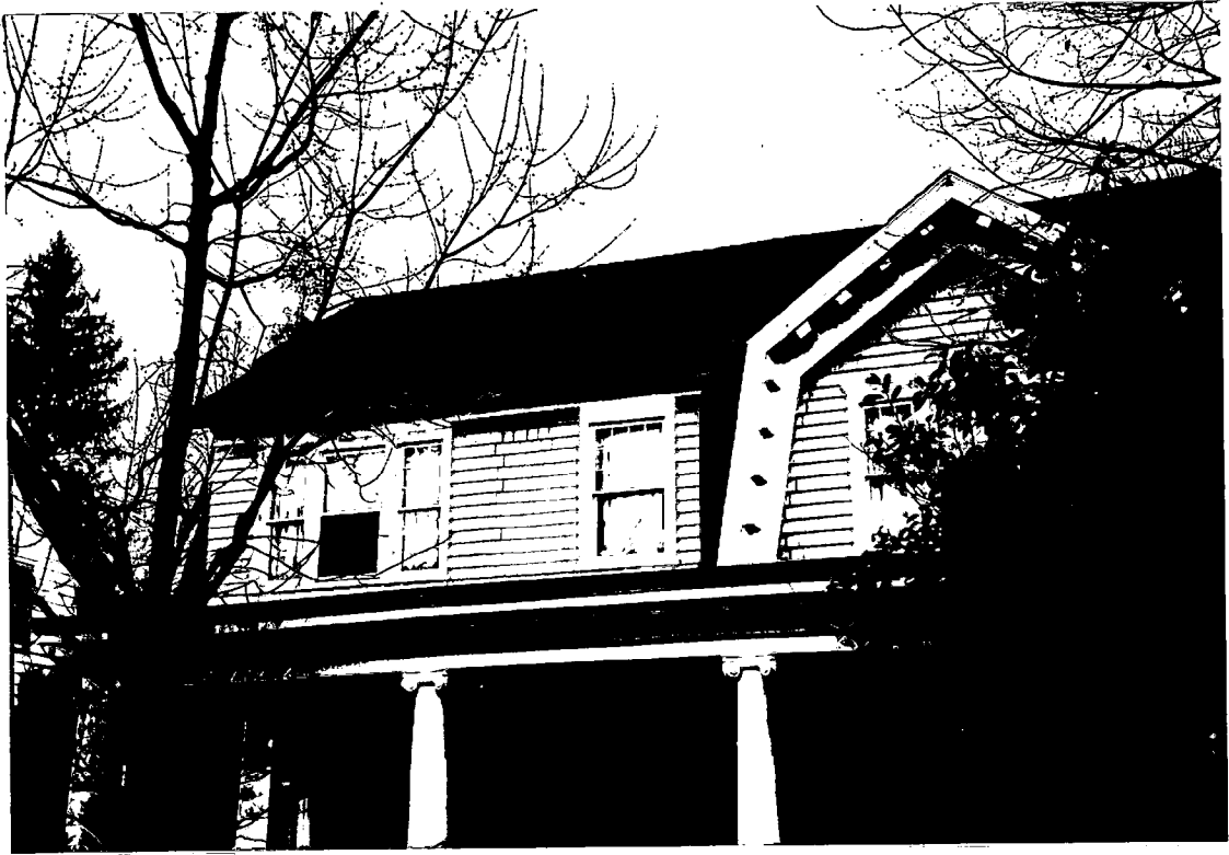
6 Hesketh Street (Above) w/ asphalt roof
