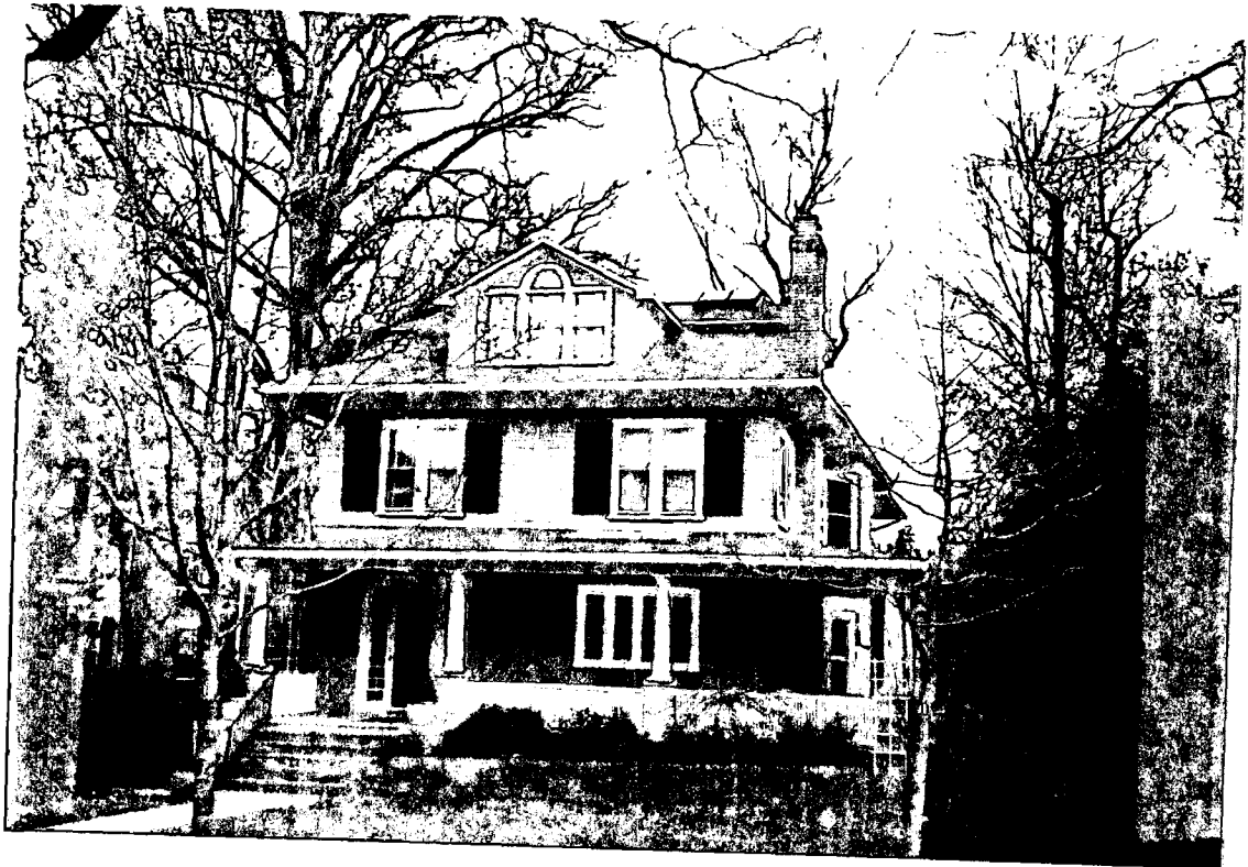
3 Hesketh Street (Above) w/ asphalt roof
