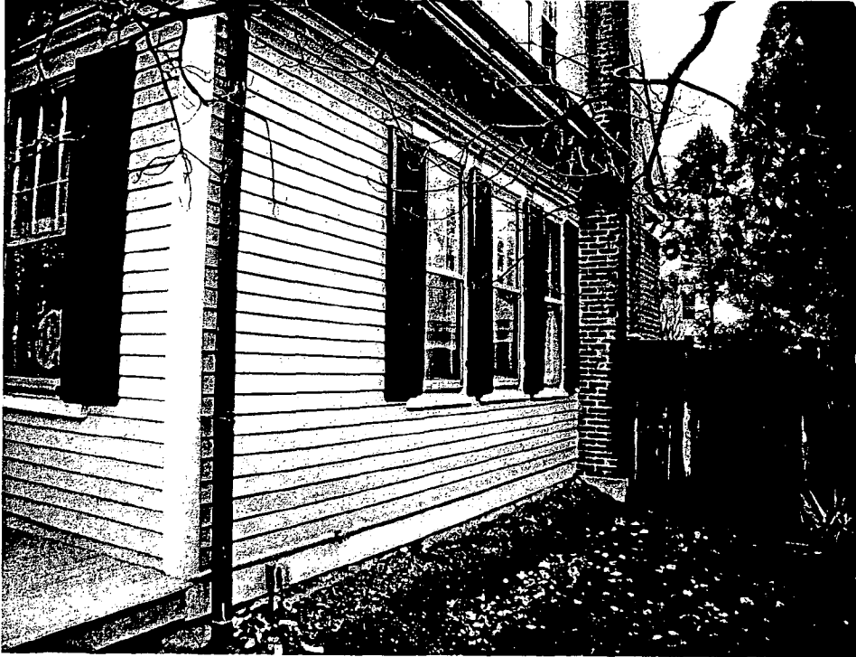
Detail: View of East Facade
