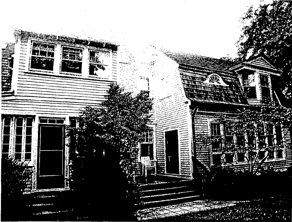
Detail: View from Northeast (Rear View) of Existing House
