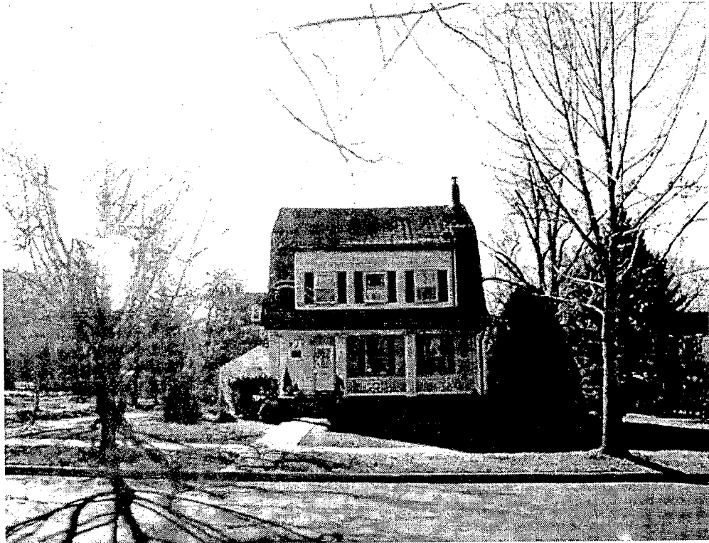
View from across the street, 14 Grafton, showing house in relation to its lot
