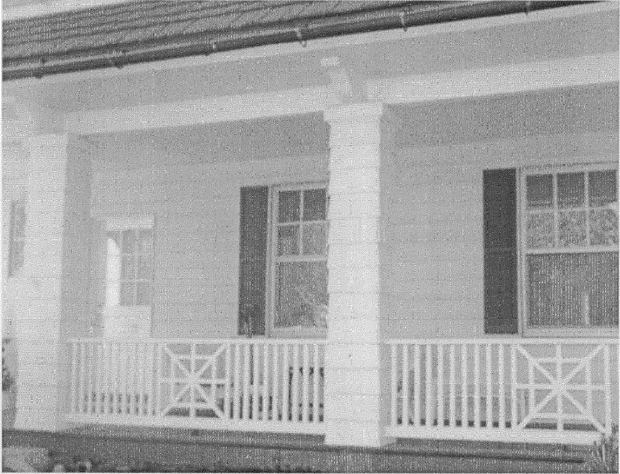
Detail of porch showing 6/1, shake-covered porch posts, and decorative railing
