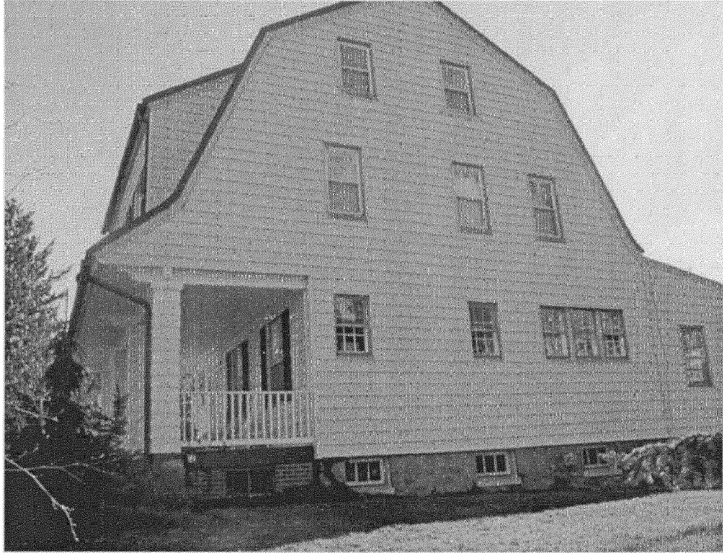
View of west wall
