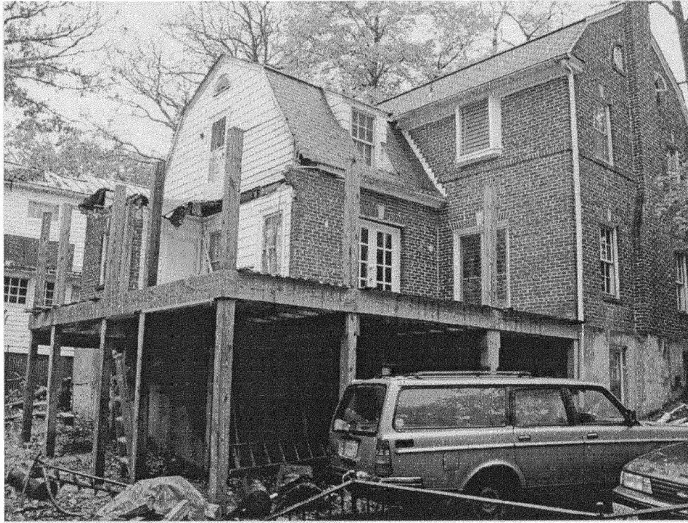
Rear of house and 1 st floor deck construction
