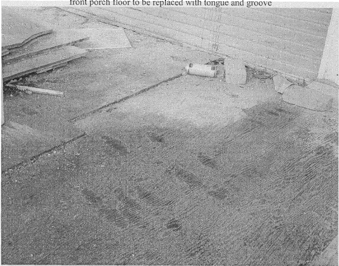
front porch floor to be replaced with tongue and groove
