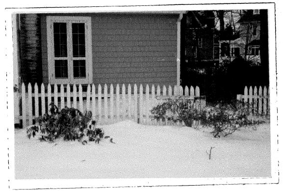
Existing fence which is in extreme disrepair. corently posts are rotted and there are rusty nails exposed. The existing fence is beyond repair.
