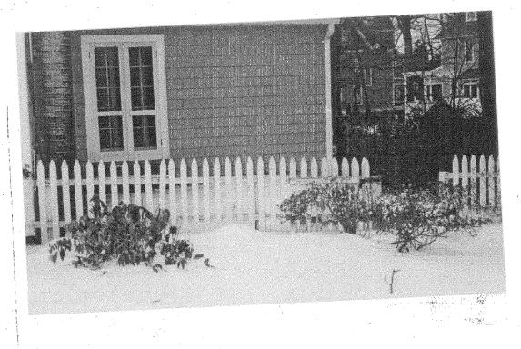
Existing fence which is in extreme disrepair. curently posts are rotted and there are rusty nails exposed. The existing fence is beyond repair.
