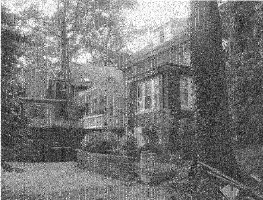
BELOW: View from southeast side
