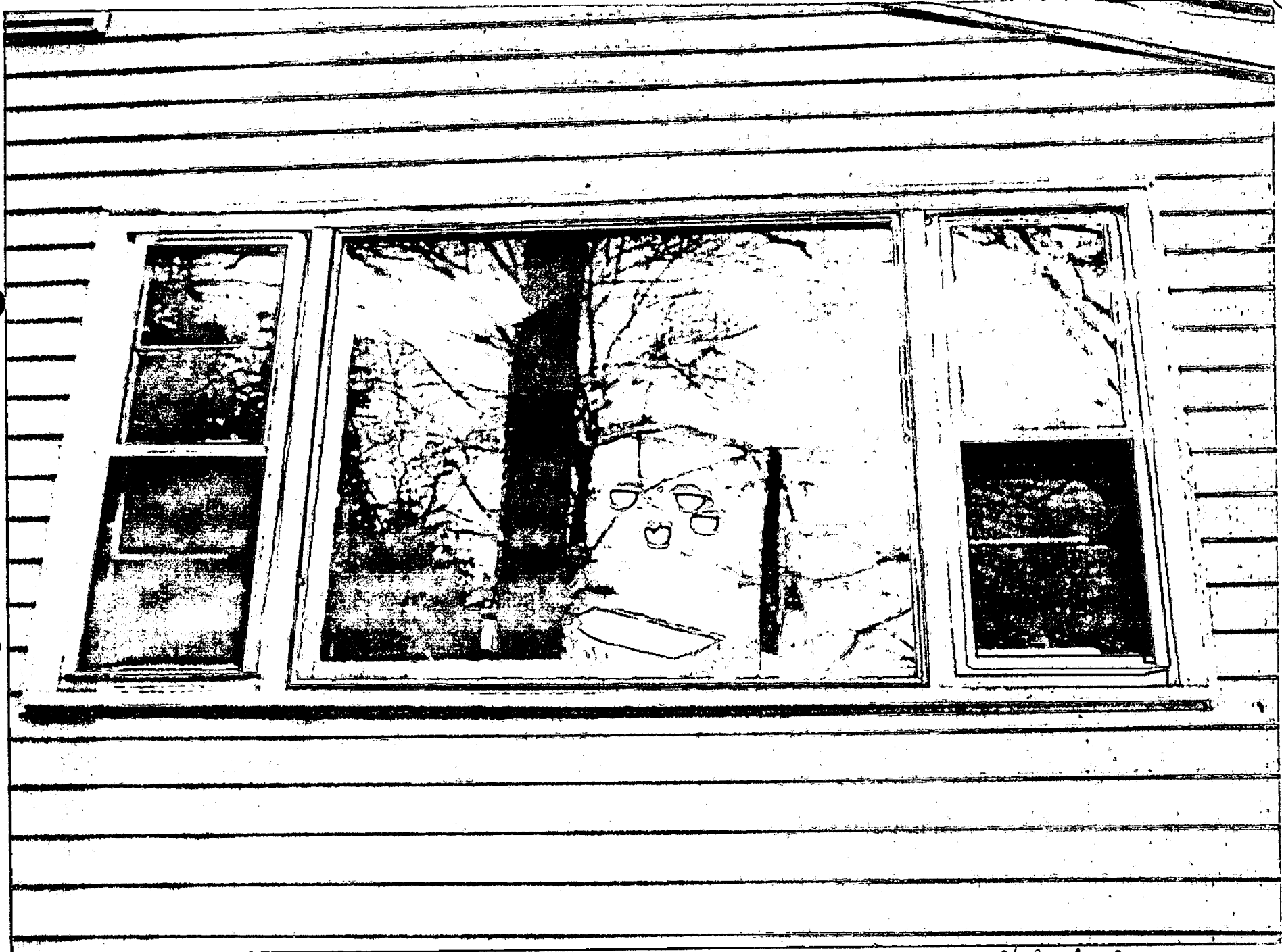
57111 Cedar Avenue. WINDOW TO BE REPLACED
