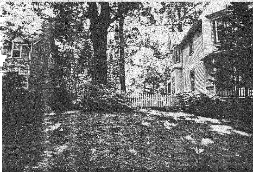
(A) VIEW FROM STREET SIDE YARD
