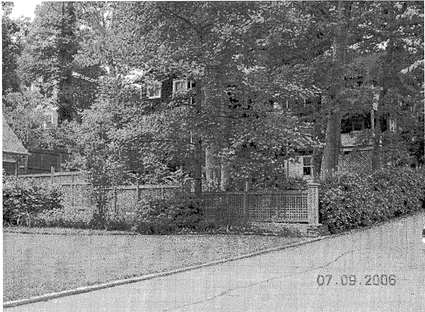
FENCE AND RETAINING WALL AT REAR PROPERTY LINE
