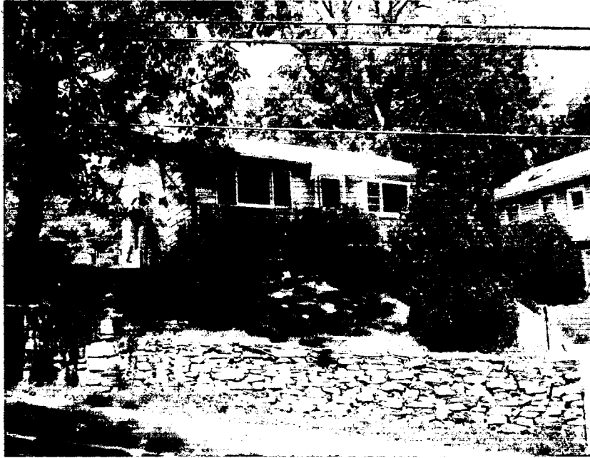
Street (Southeast) Elevation
