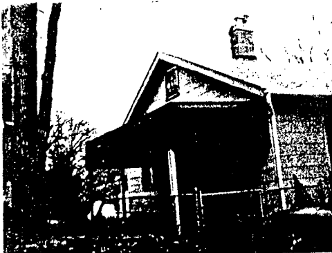
North West Facade
