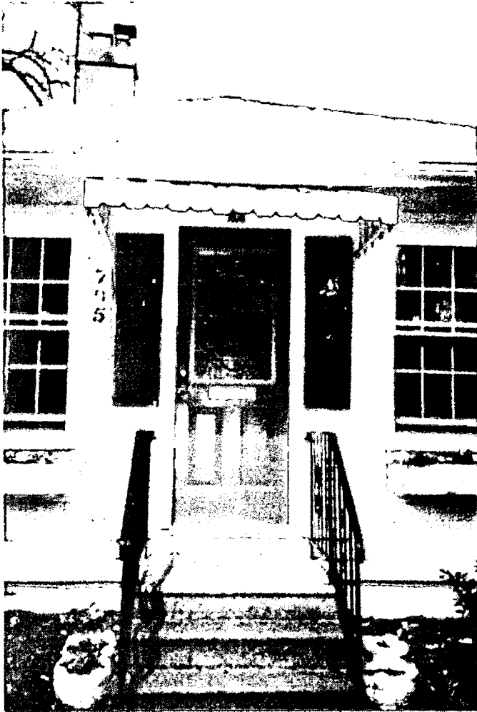
Aluminum awning to be replaced with wood awning
